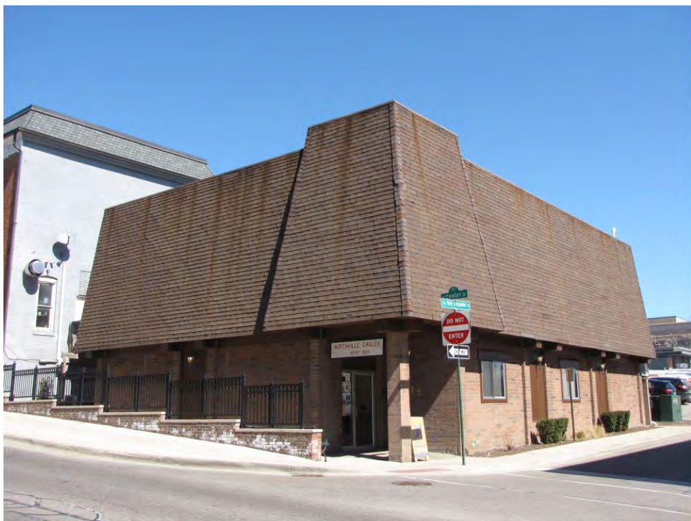
Center South 113_Looking Northeast
