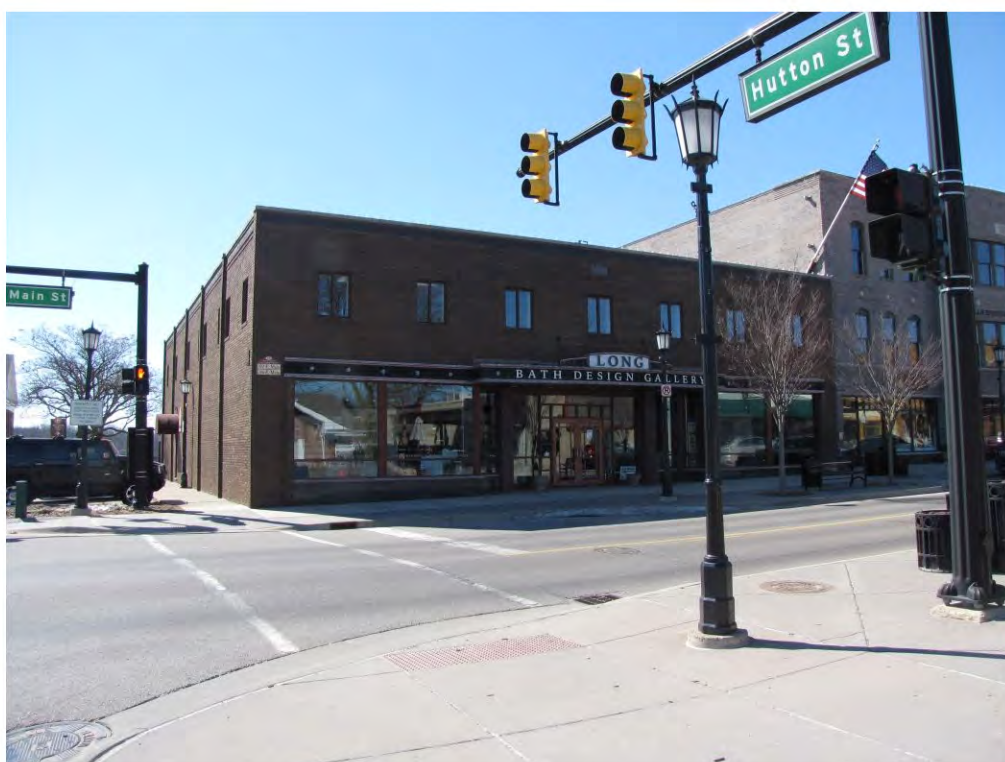
Main East 190_Looking Southwest
