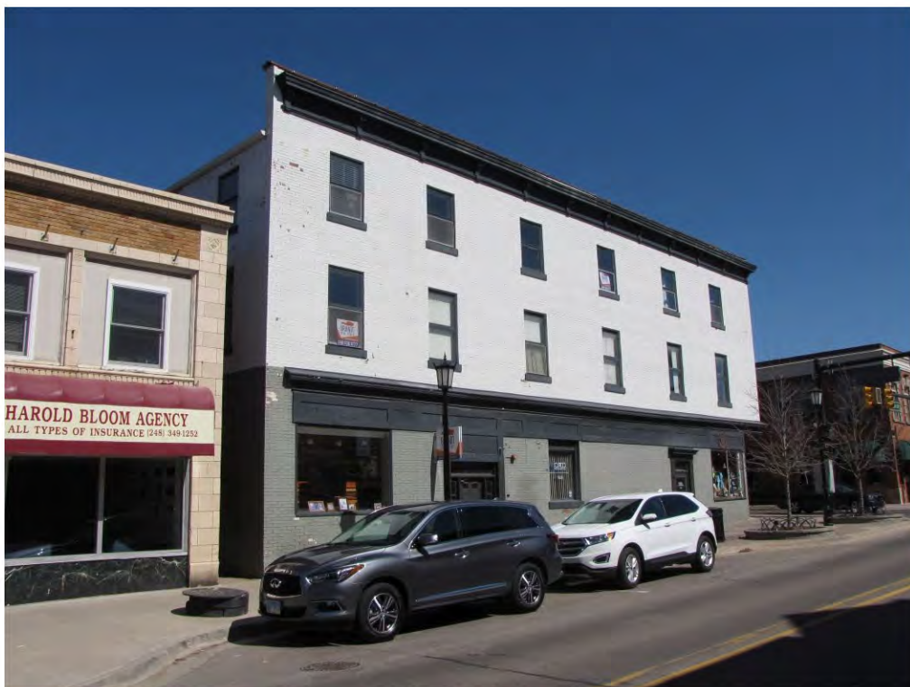
Center North 101-103 and Main West 102-106_Looking West
