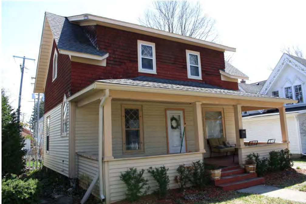
Wing North 212_Looking Southeast
