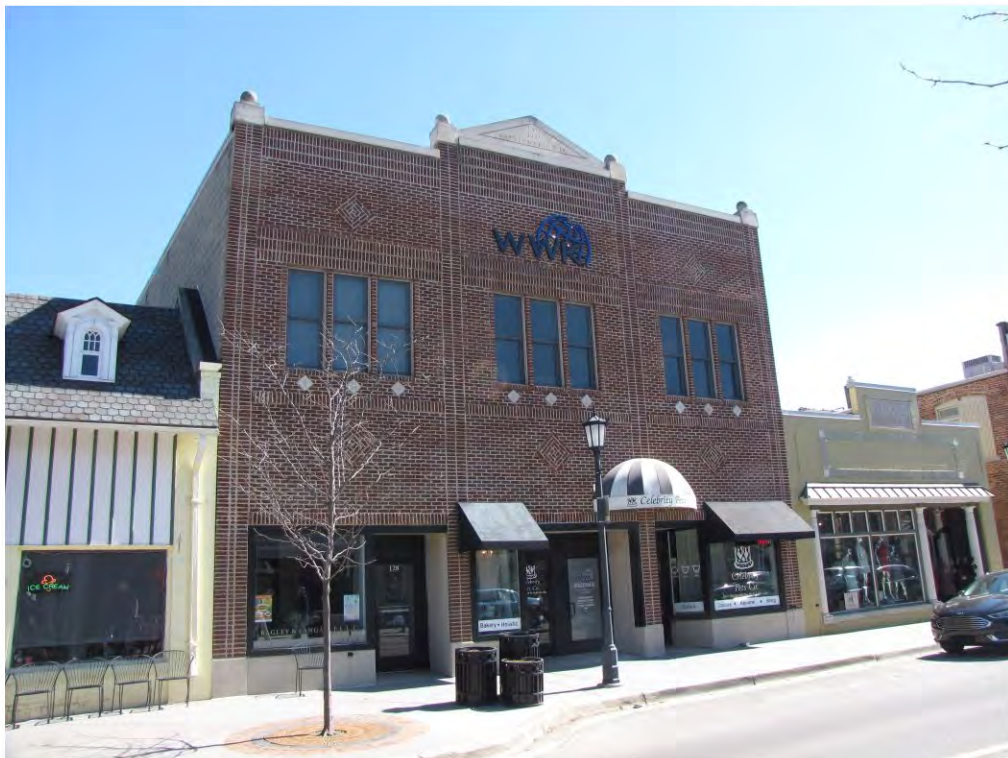
Center North 124-128_Looking Northeast
