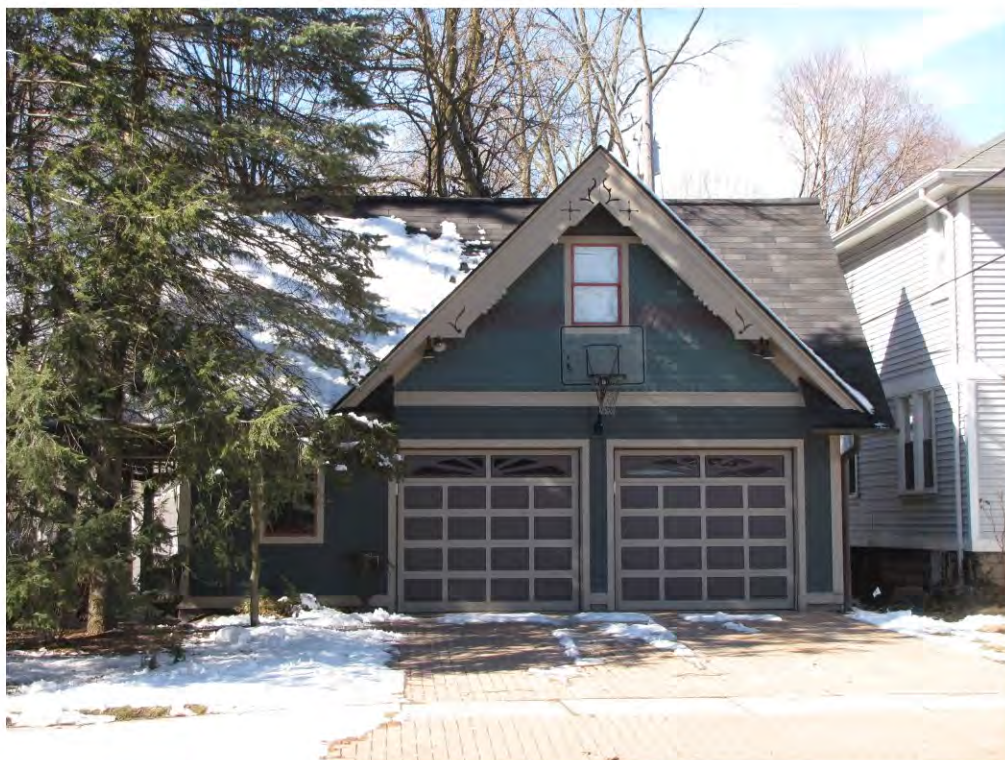
Dunlap West 504, Garage_Looking West
