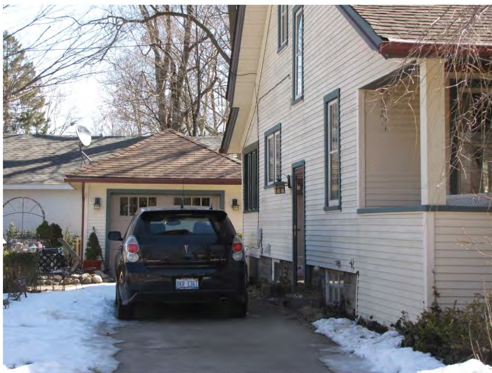
Linden 118, Garage_Looking East
