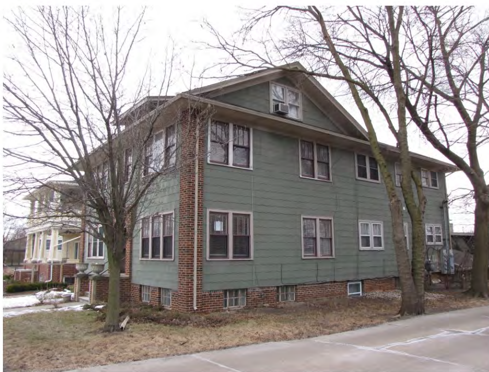
Main East 430_Looking Southeast
