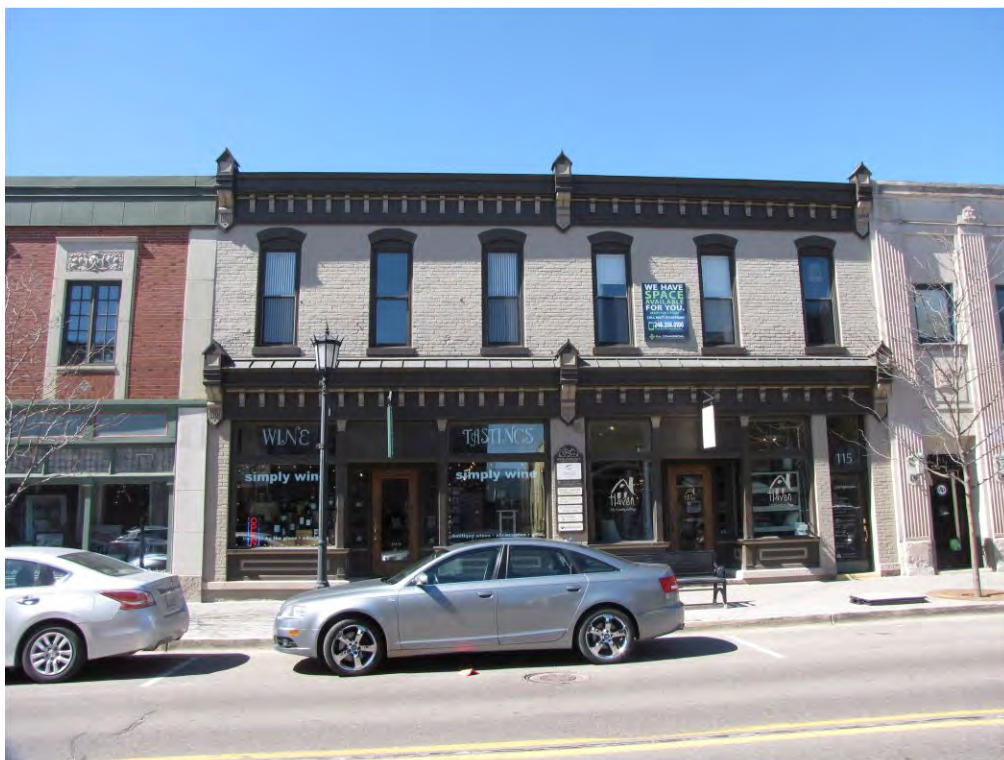
Center North 109-115_Looking West
