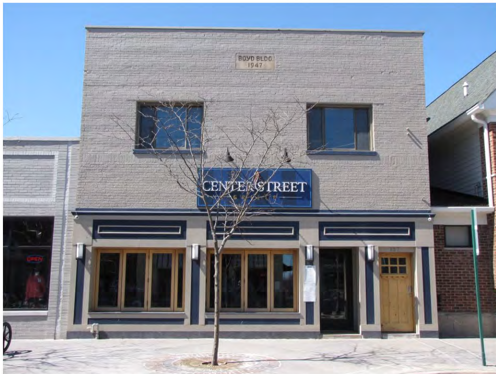
Center North 135-137_Looking West
