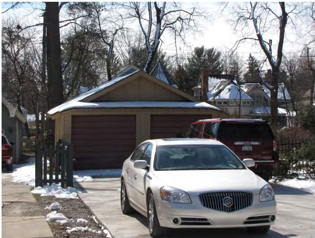
Main West 547, Garage_Looking South
