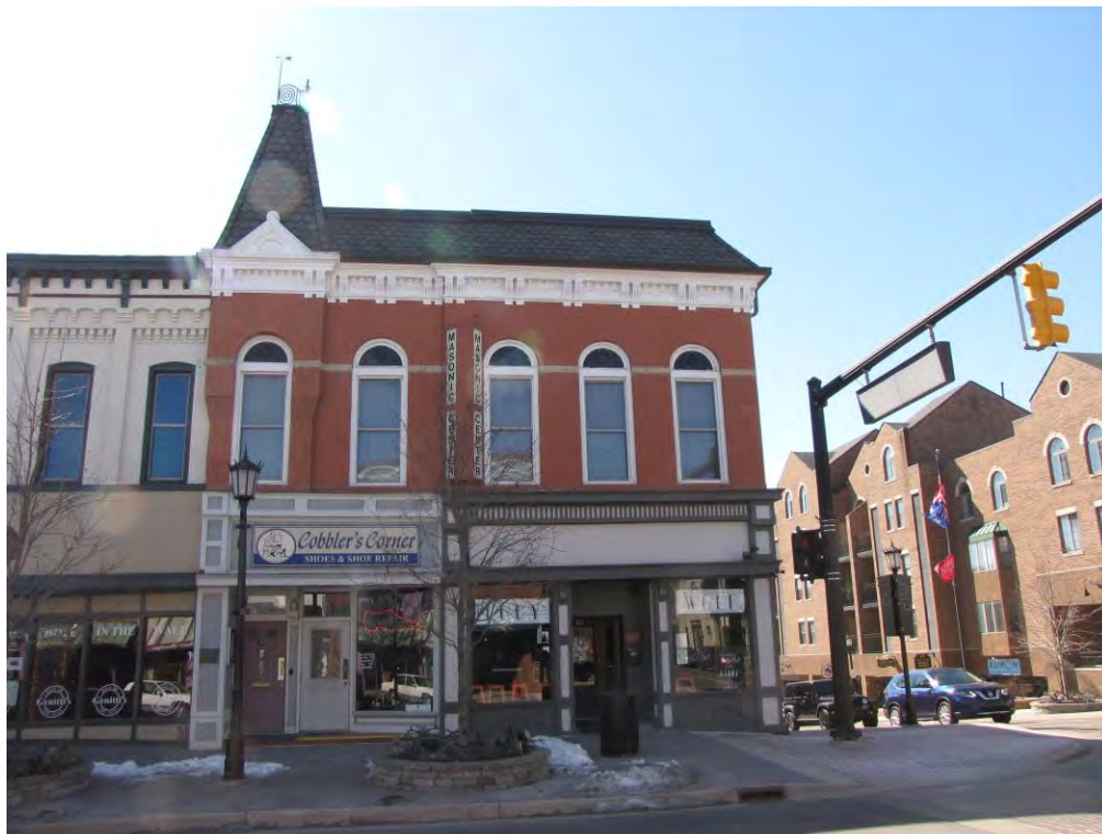
Main East 102-106 and Center South 113_Looking South
