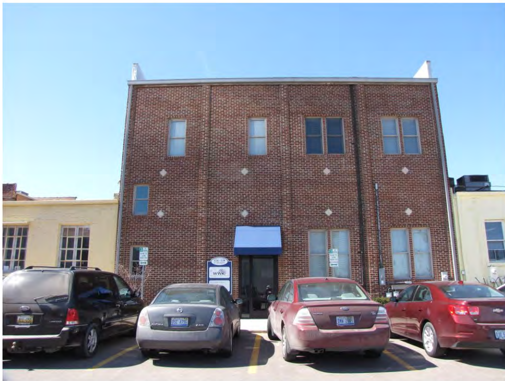
Center North 124-128_Looking Southeast
