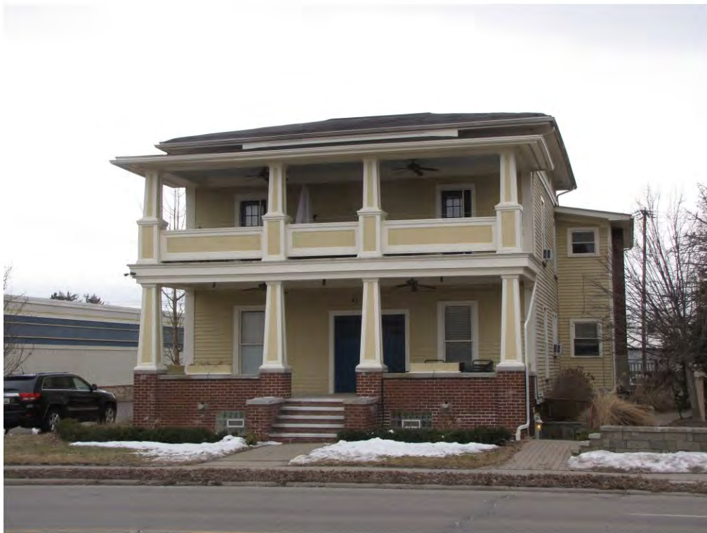
Main East 450_Looking Southeast
