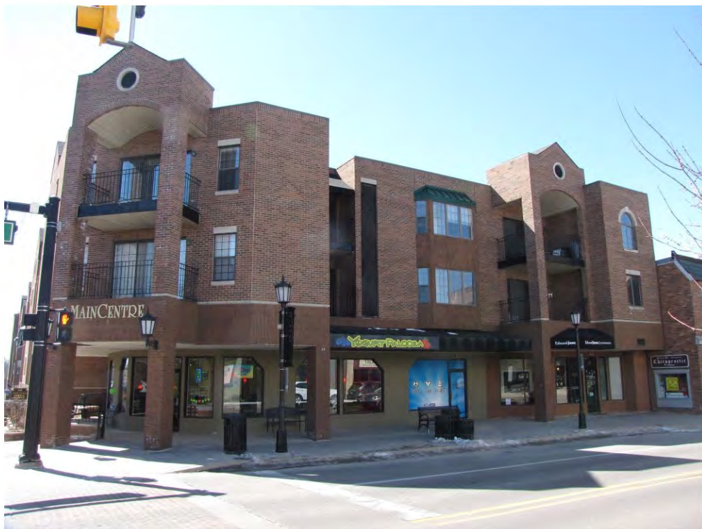
MainCentre 150_Looking Southwest
