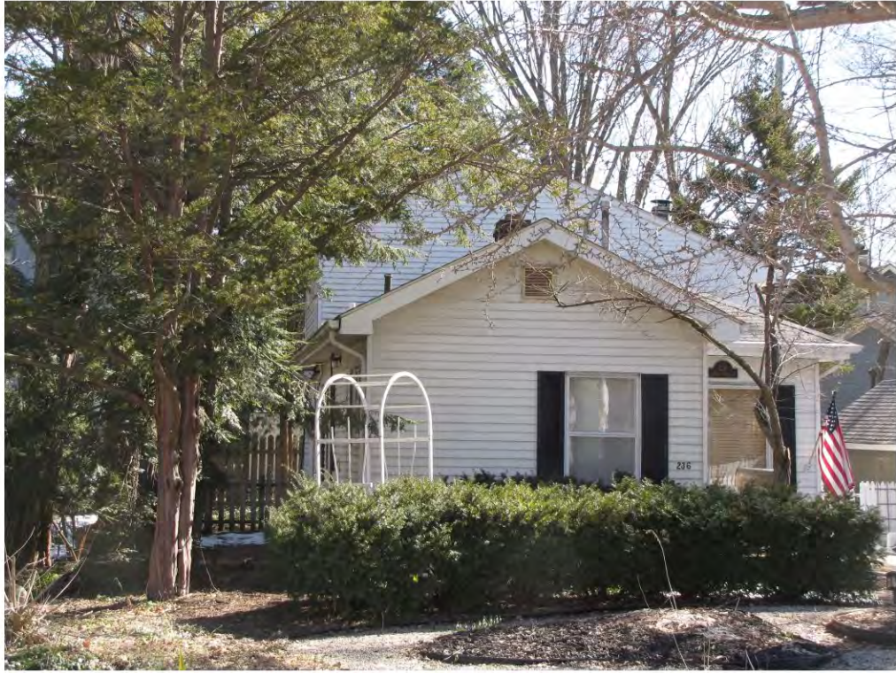
West 236-Looking East
