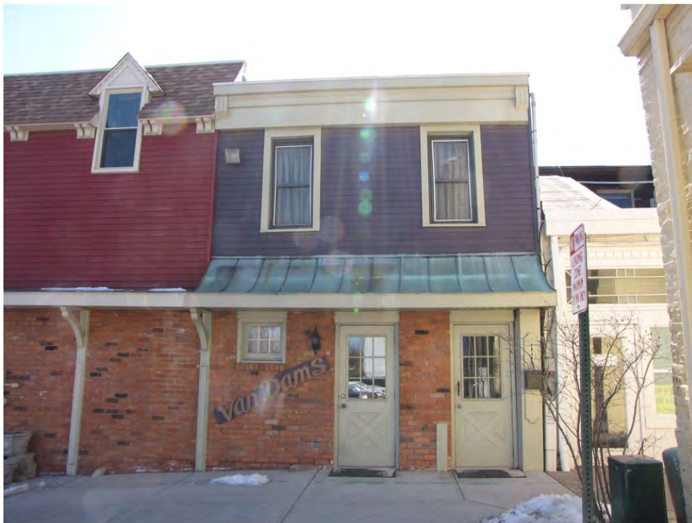
Main East 111_Looking South
