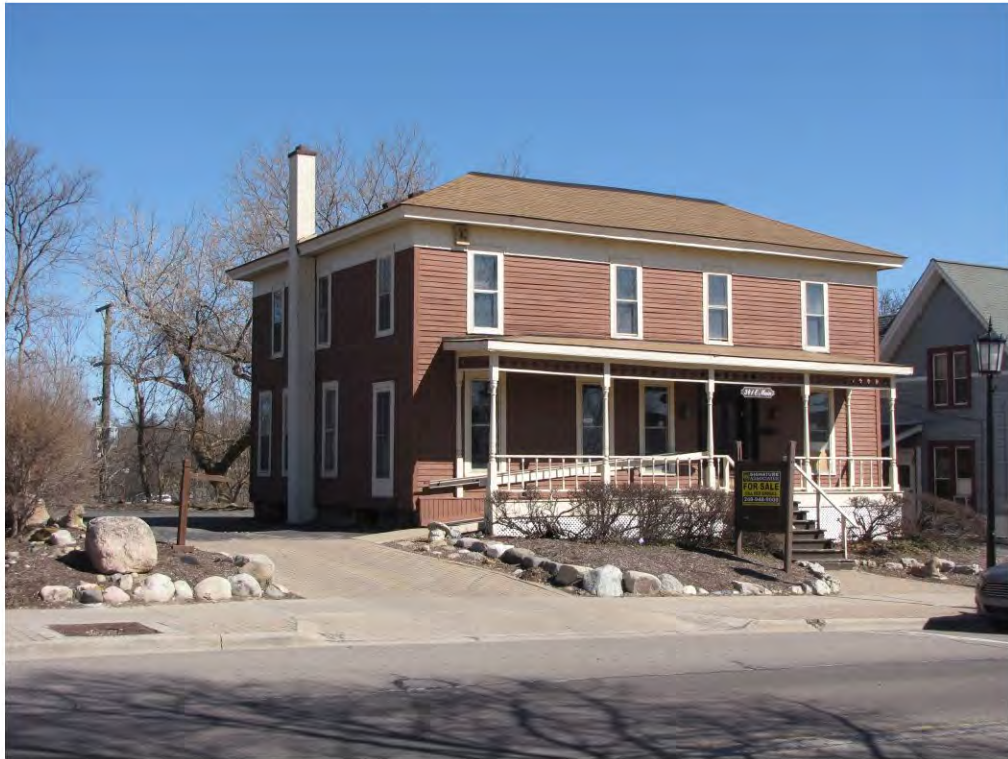
Main East 341_Looking Northeast
