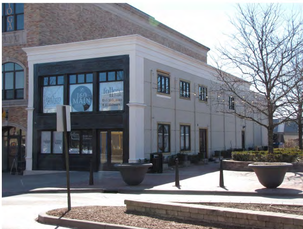
Main East 160_Looking Southeast
