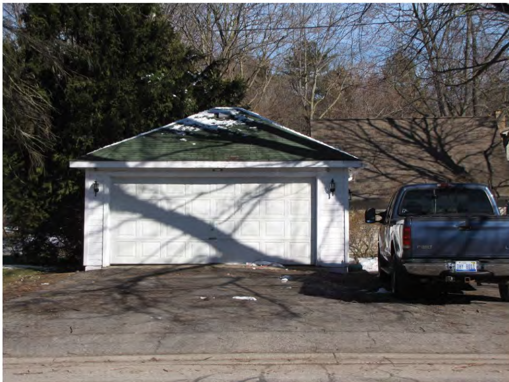
Rogers North 101, Garage_Looking North
