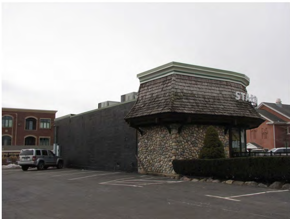
Main East 302_Looking Southwest
