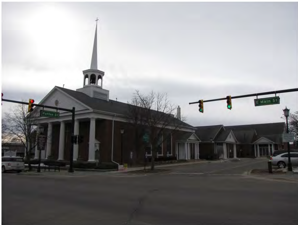
Main East 200_Looking Southeast
