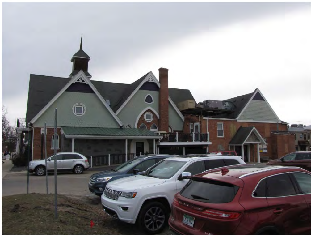
Center North 145-Looking East
