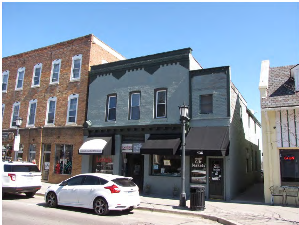
Center North 136-142_Looking Northeast
