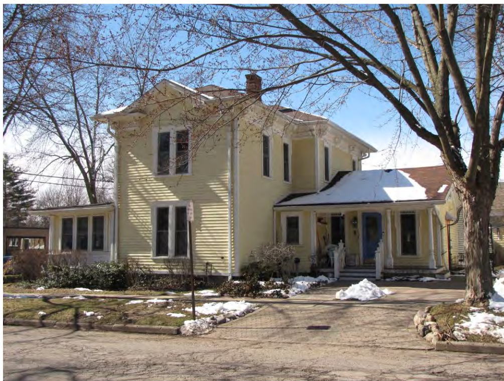
Main West 502_Looking Northeast
