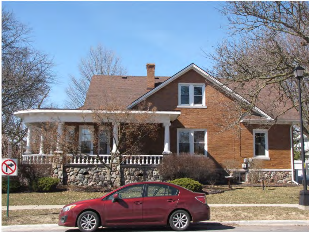
Main West 302_Looking West
