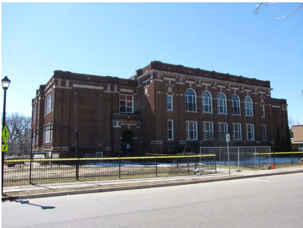
Main West 411_Looking South
