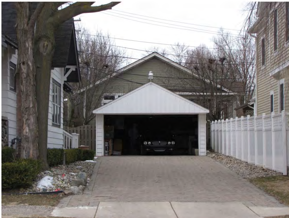
Wing North 111, Garage_Looking West
