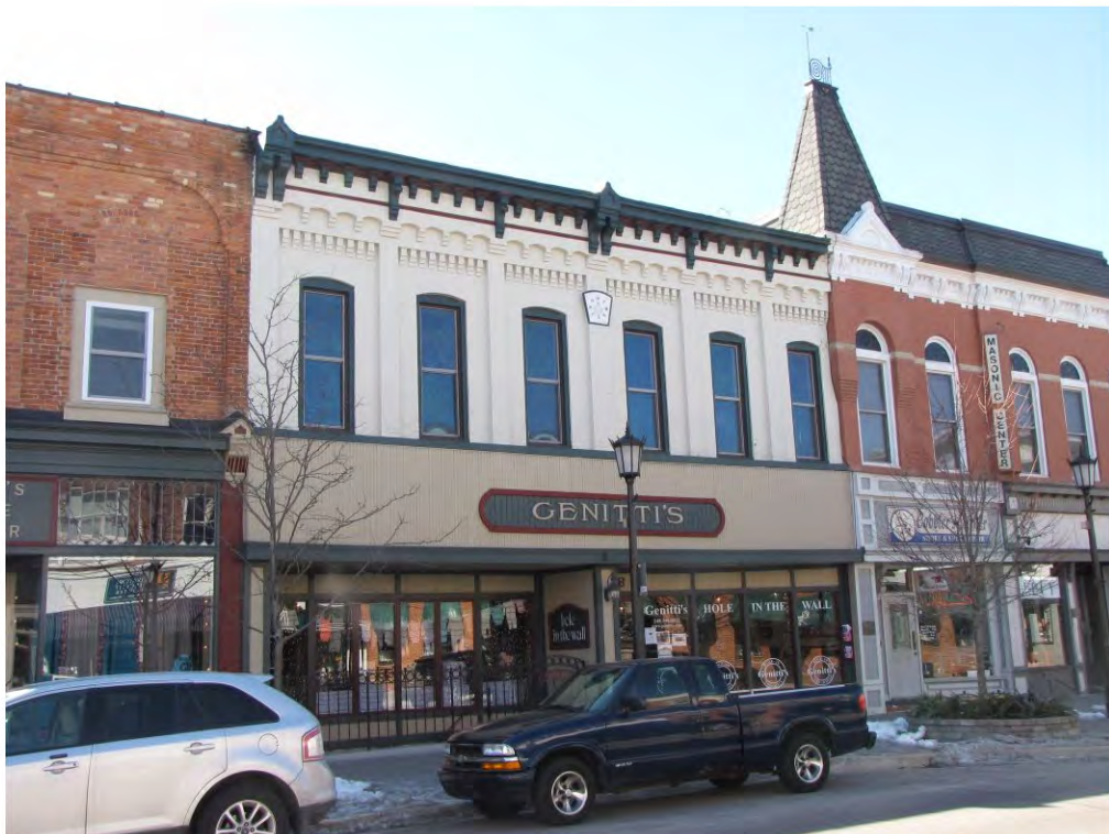
Main East 108-110_Looking Southeast
