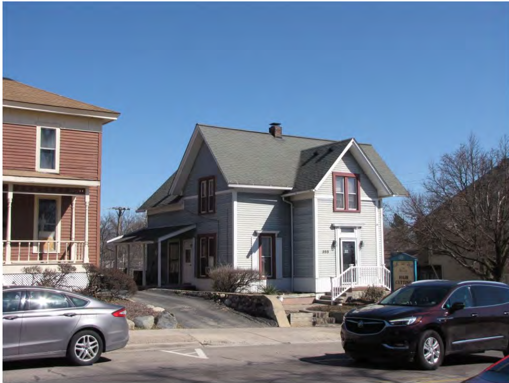
Main East 355_Looking Northeast
