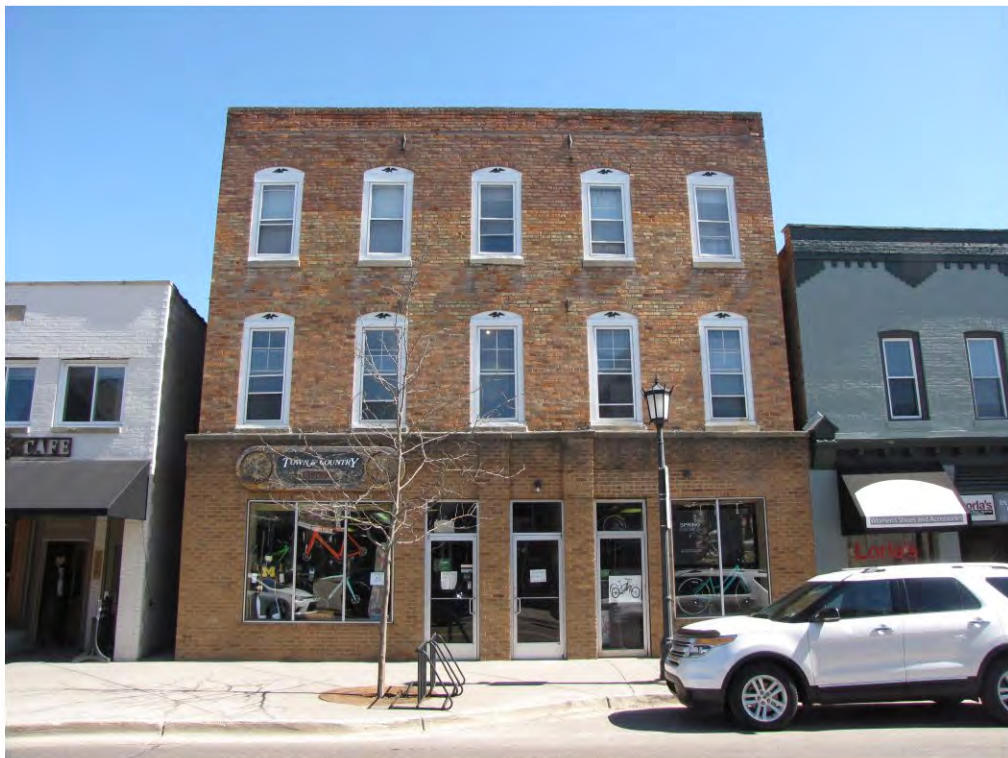
Center North 144-148_ Looking East
