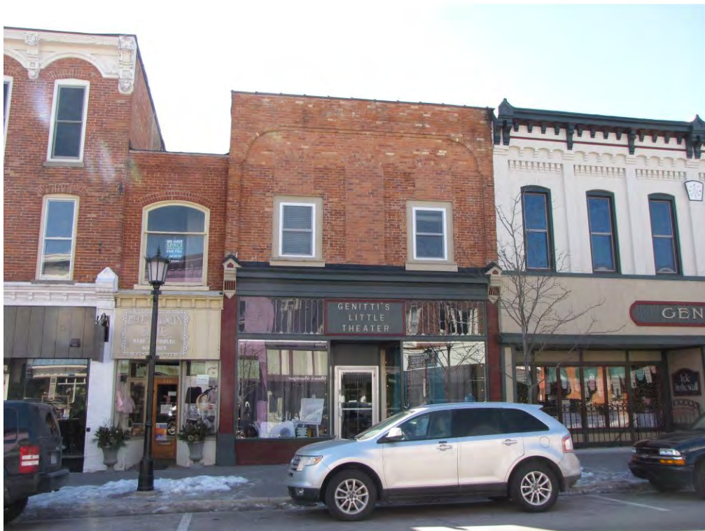
Main East 112_Looking South
