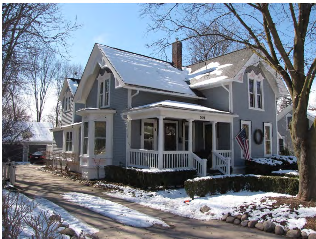
Main West 521_Looking Southwest
