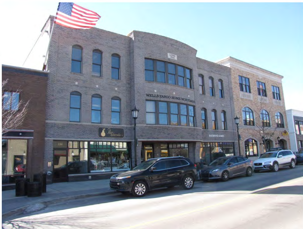
Main East 182-186_Looking Southwest
