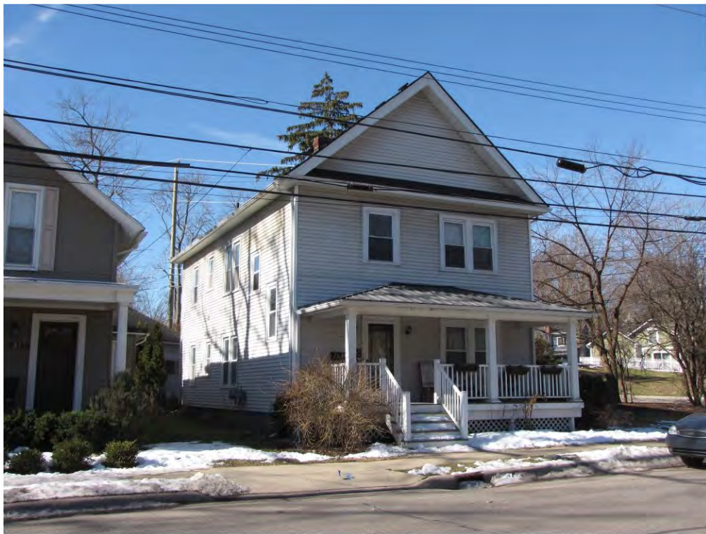
Randolph 319-321_Looking Southwest
