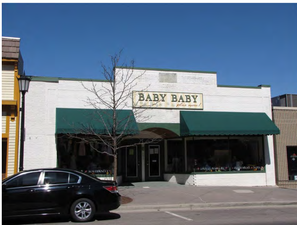
Main East 153_Looking Northeast
