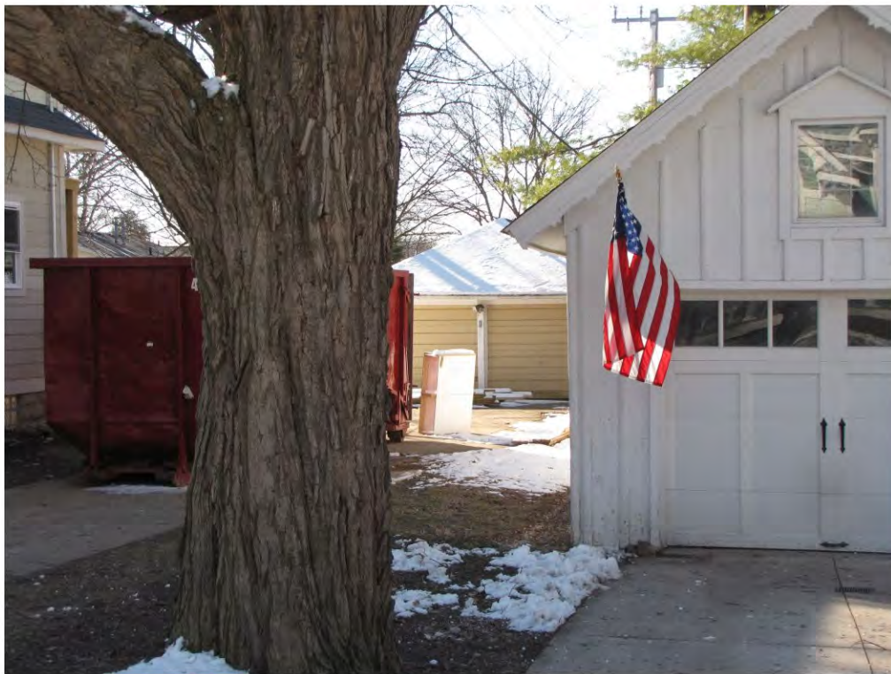
Cady West 511, Garage_Looking South
