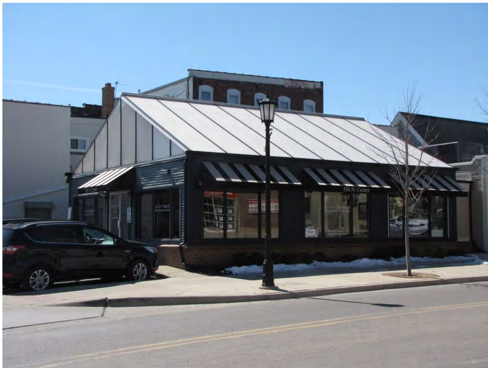
Center North 156_Looking Southeast
