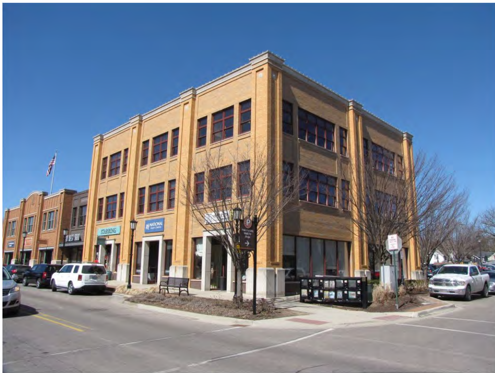
Main West 114-126_Looking Northwest
