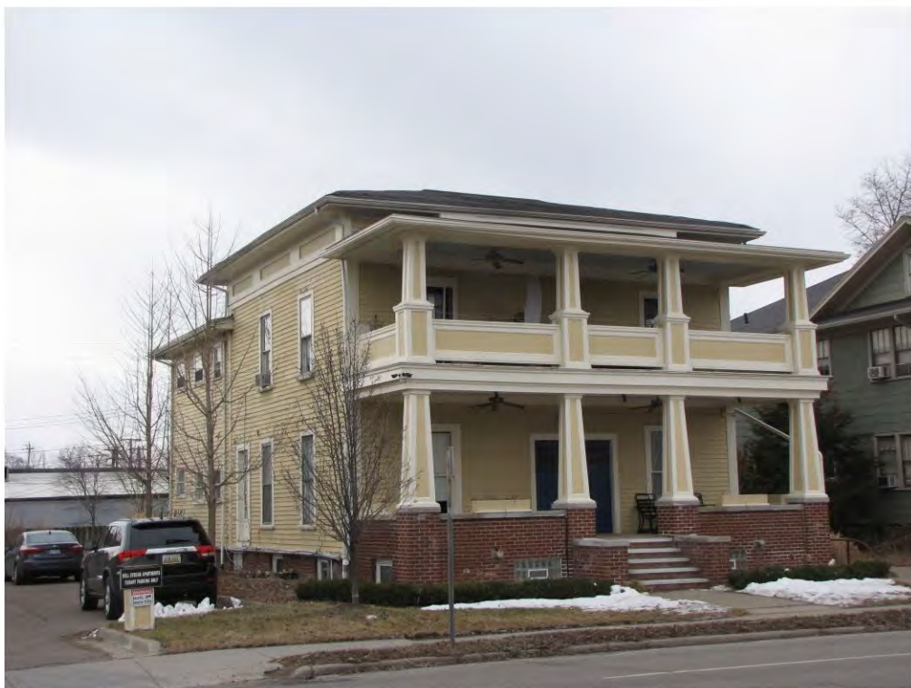
Main East 450_Looking Southwest
