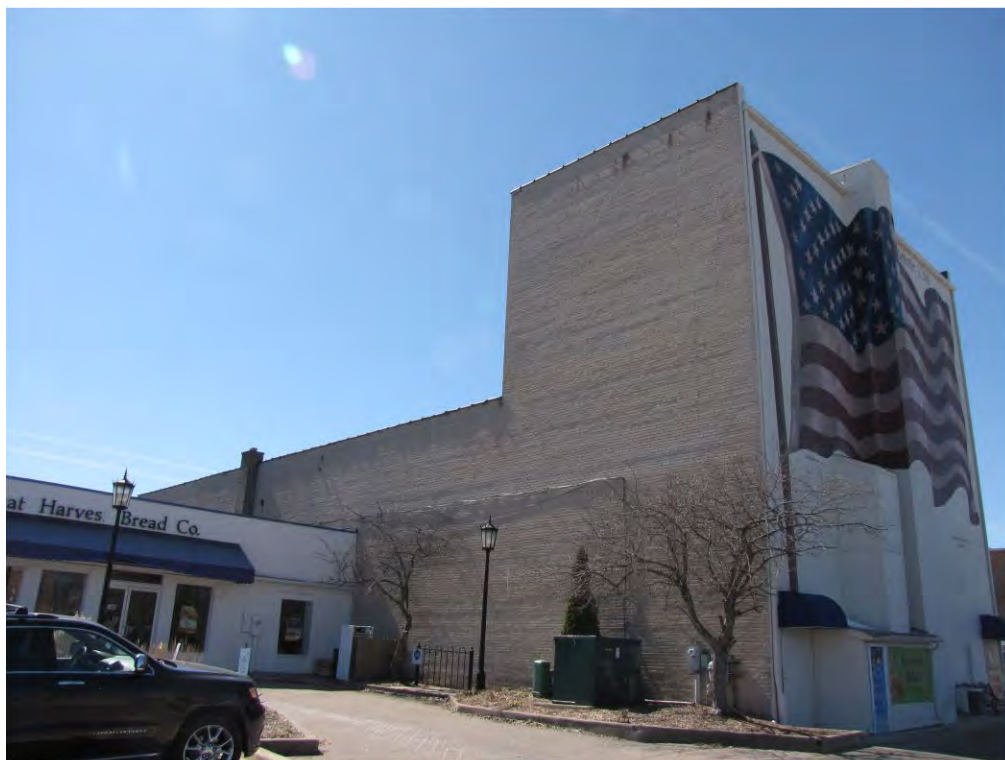
Main East 135-137_Looking Southwest
