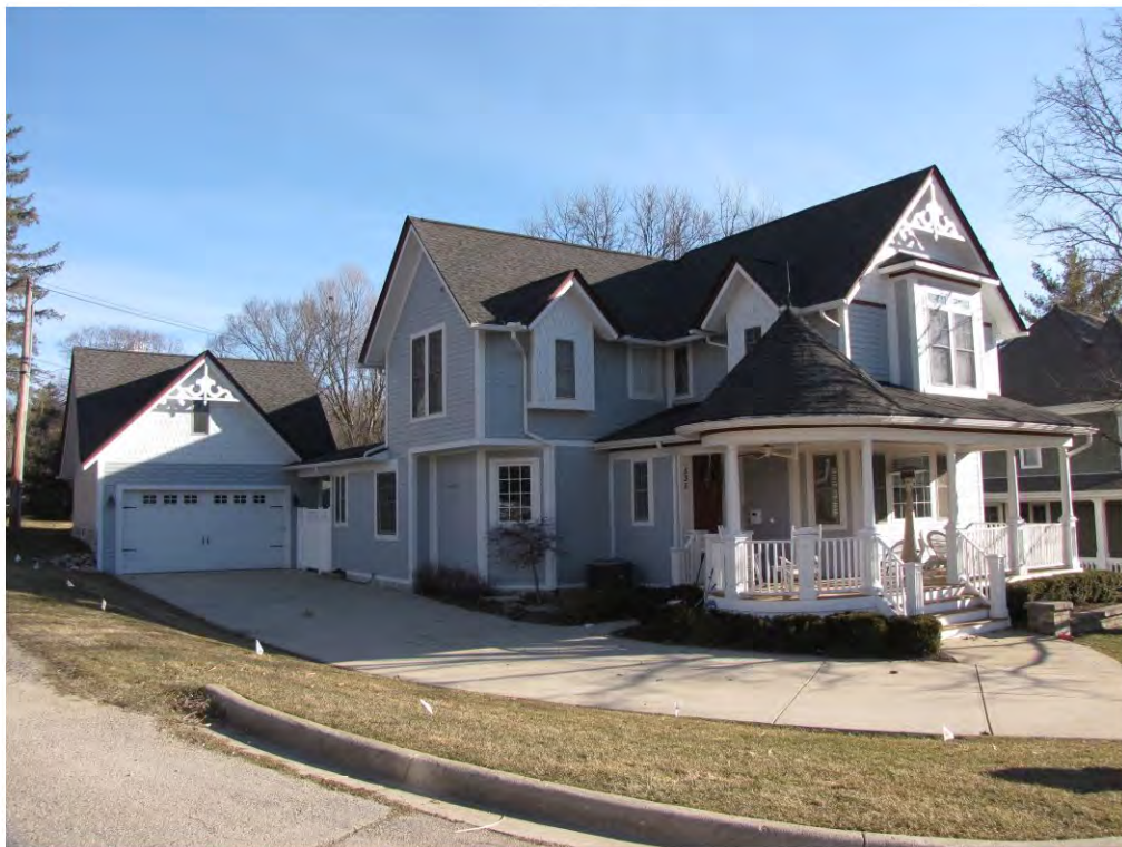
Linden Court 535_Looking Northeast
