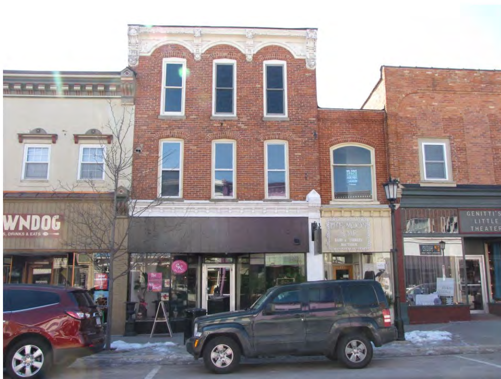
Main East 118_Looking South
