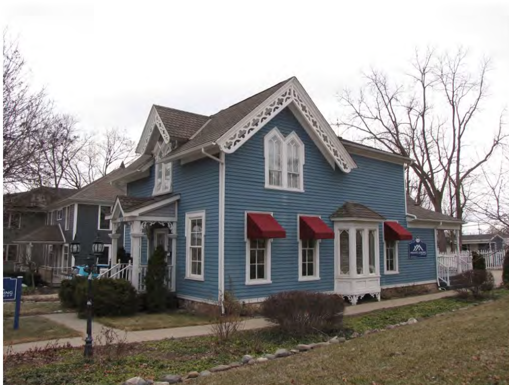
Main East 410_Looking Southeast
