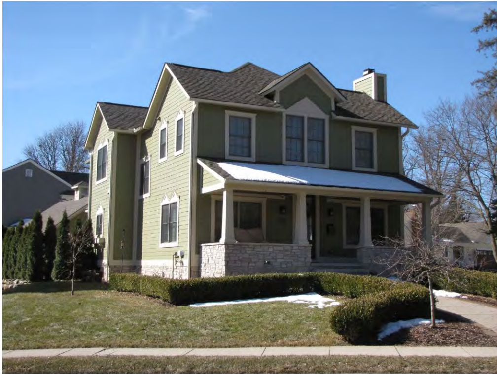
Randolph 413_Looking Southwest
