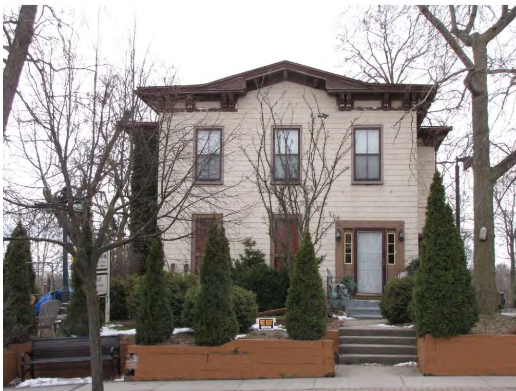
Main East 342_Looking South
