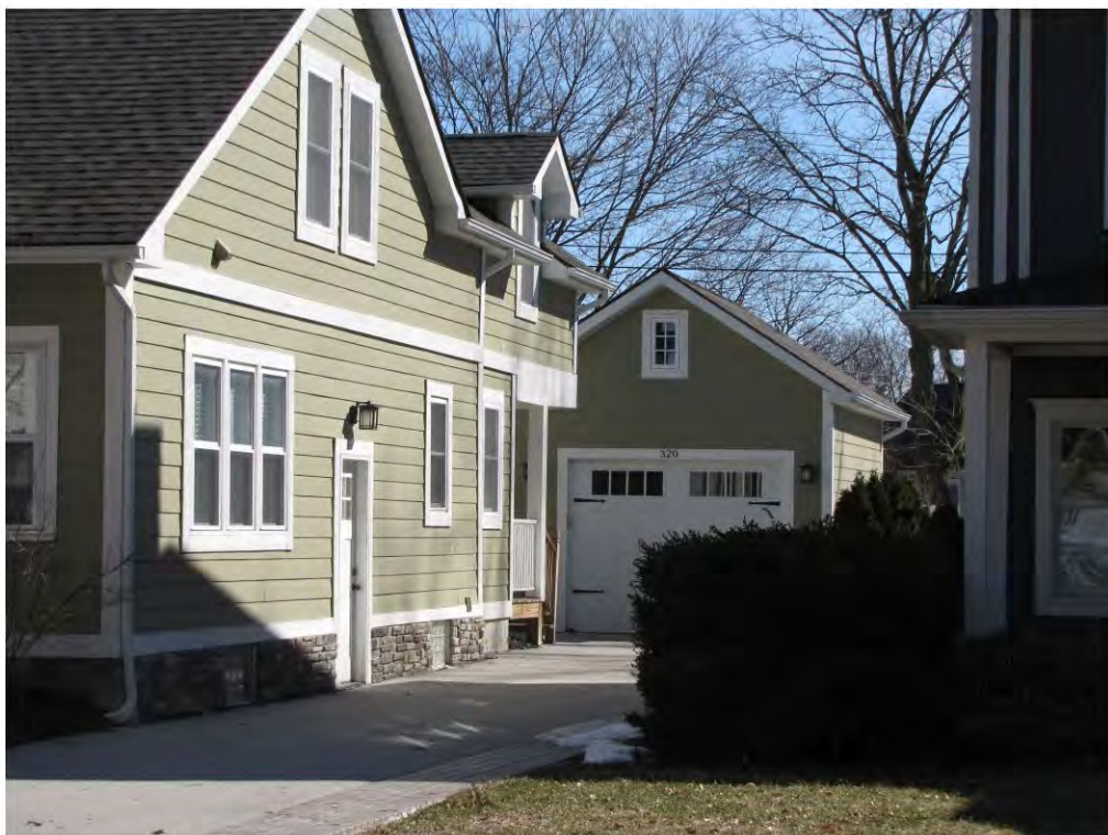
Linden 320, Garage_Looking East
