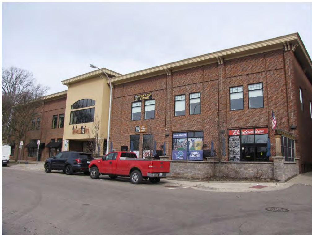
Main West 133_Looking Northwest
