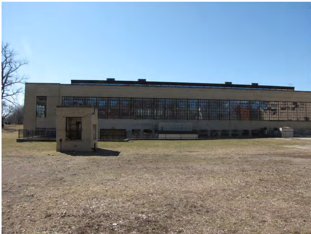
Main East 235_Looking South
