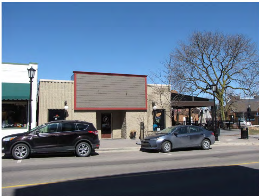
Main East 157_Looking Northeast
