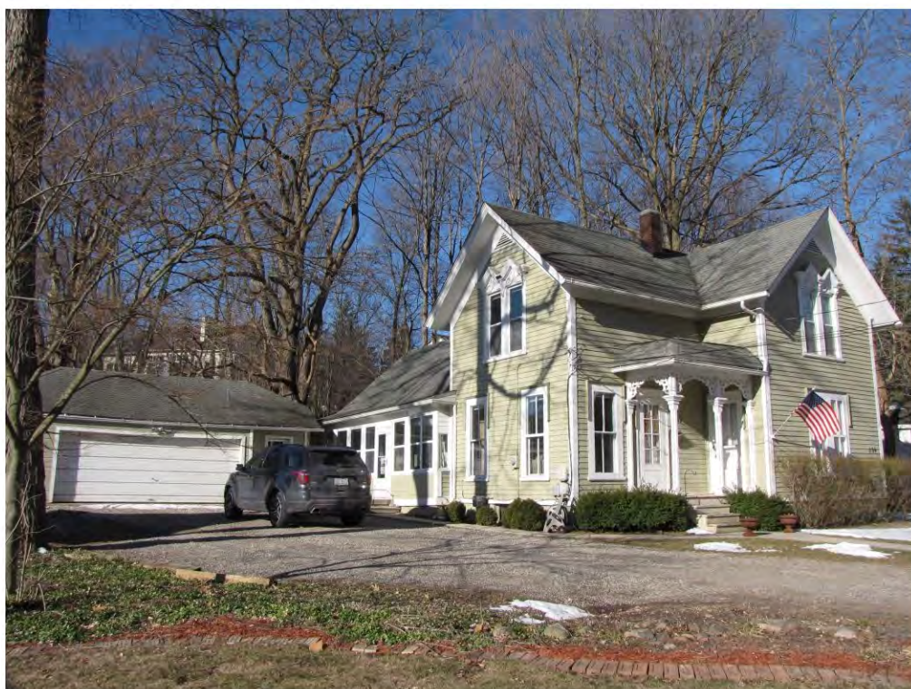
Randolph 537-539_Looking Southwest
