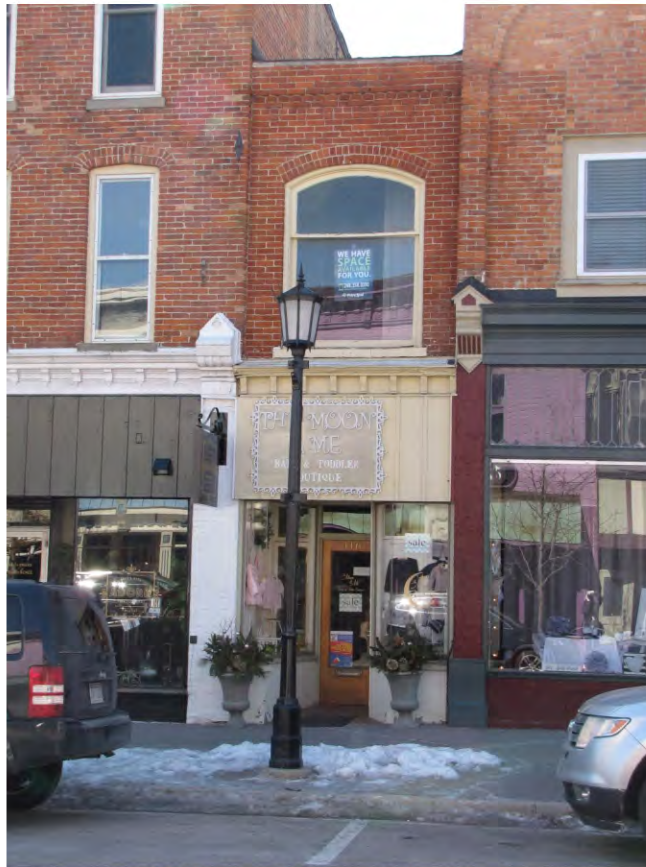
Main East 116_Looking South
