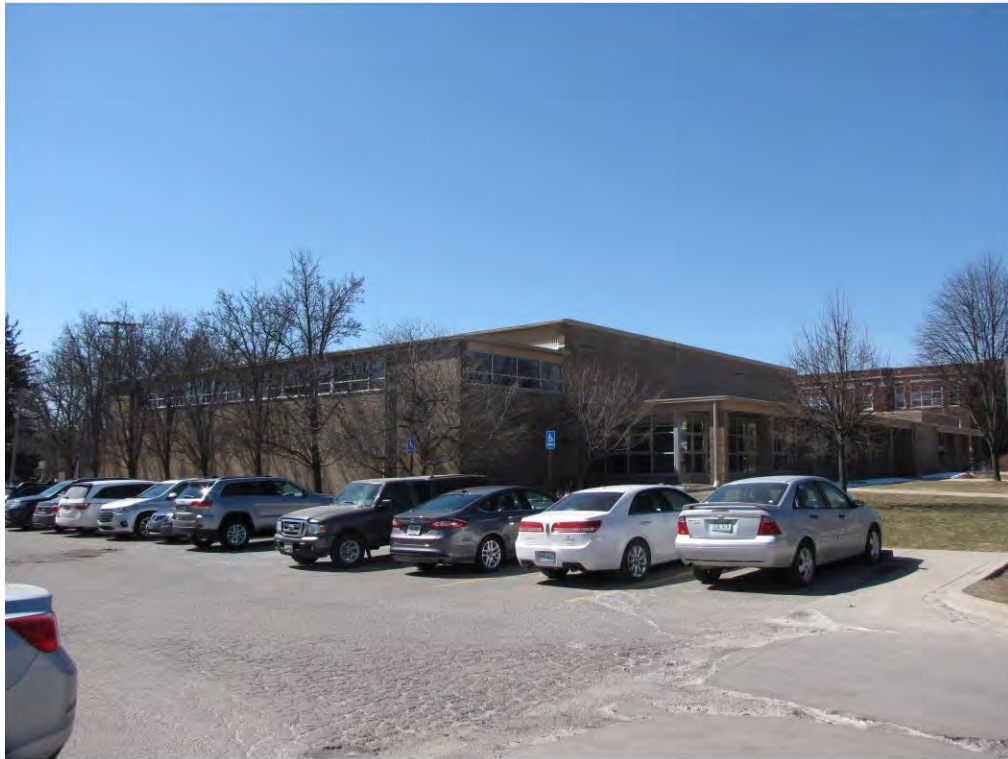
Main West 303_Looking Southwest
