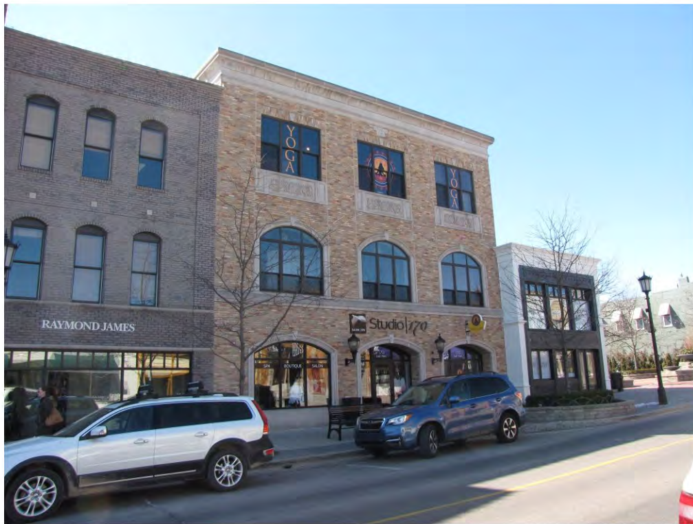
Main East 170_Looking Southwest
