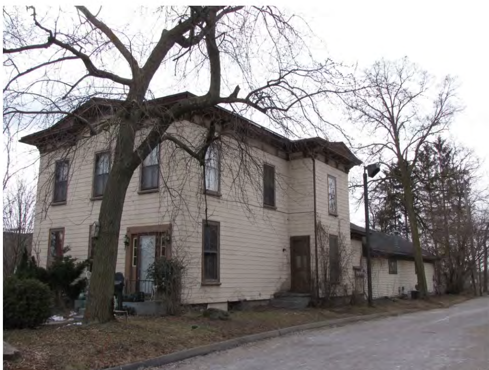
Main East 342_Looking Southeast
