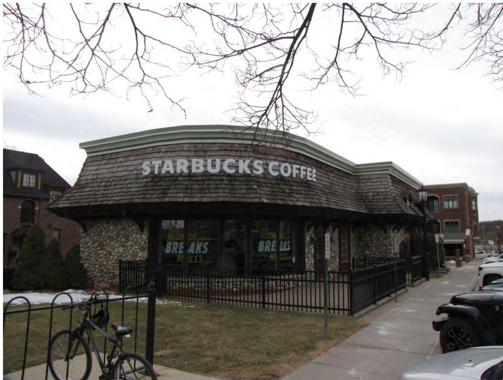
Main East 302_Looking South
