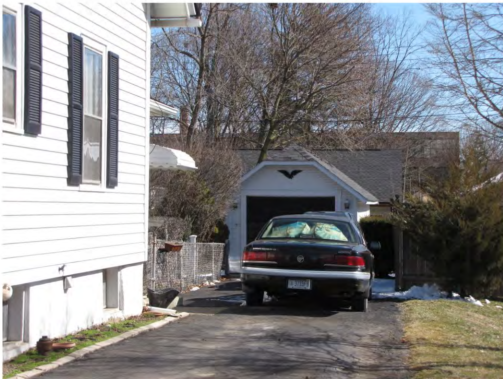
Rogers South 117, Garage_Looking East
