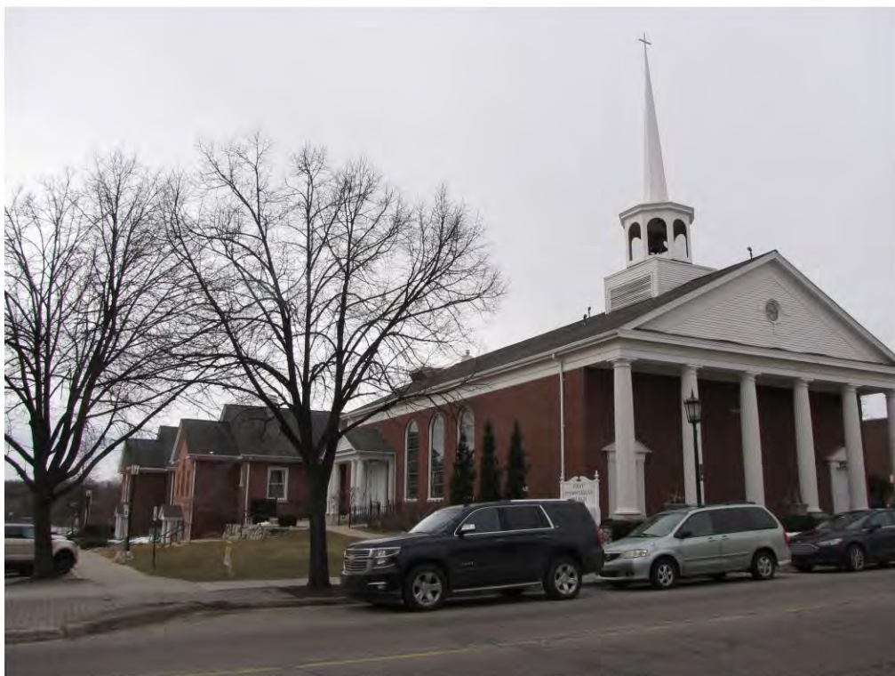
Main East 200_Looking Southwest
