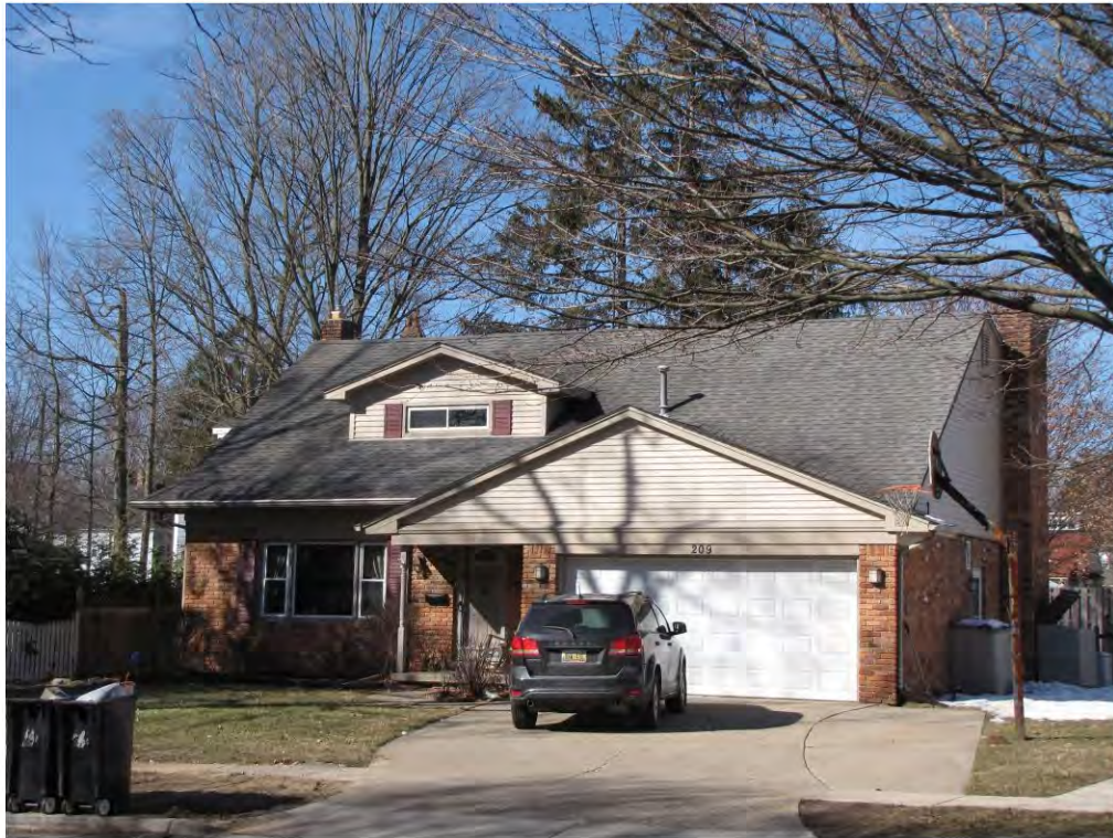
Wing North 209_Looking Southwest
