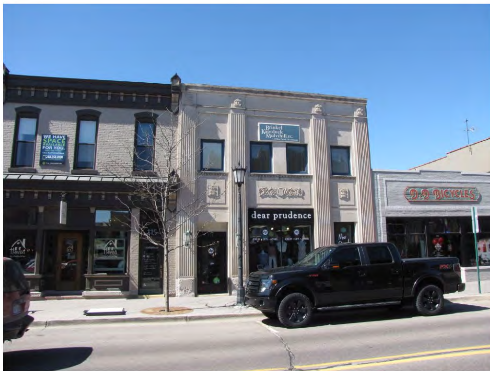
Center North 119_Looking Northeast
