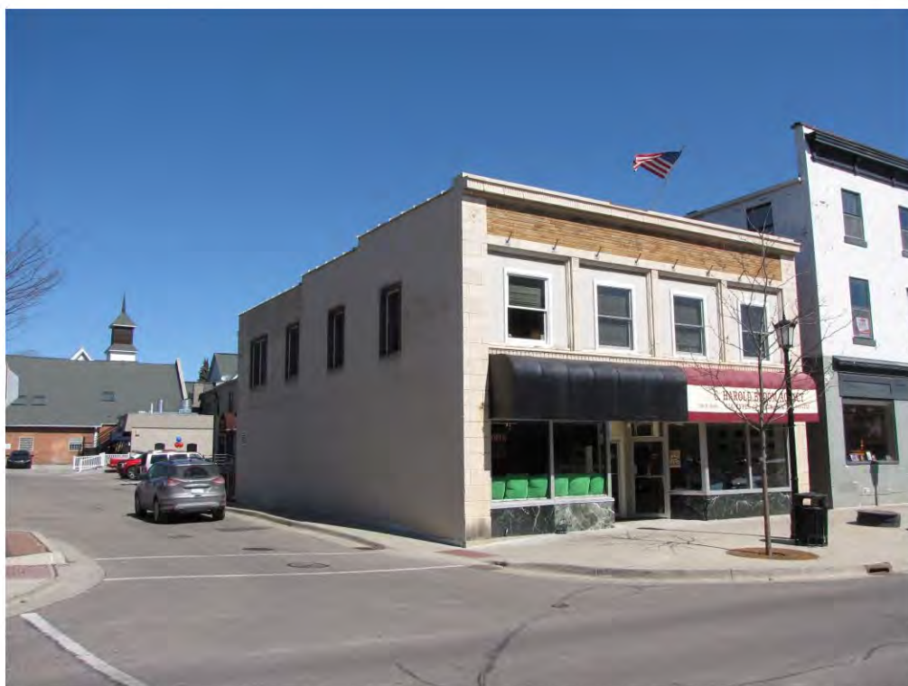
Main West 108-112_Looking Northeast
