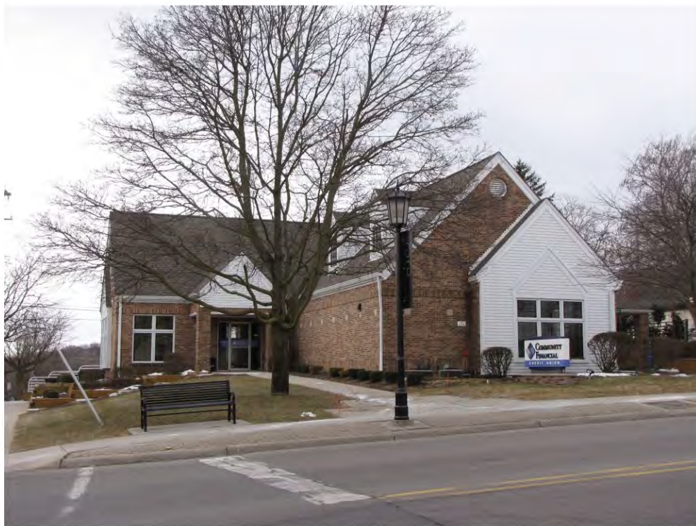
Main East 400_Looking Southwest
