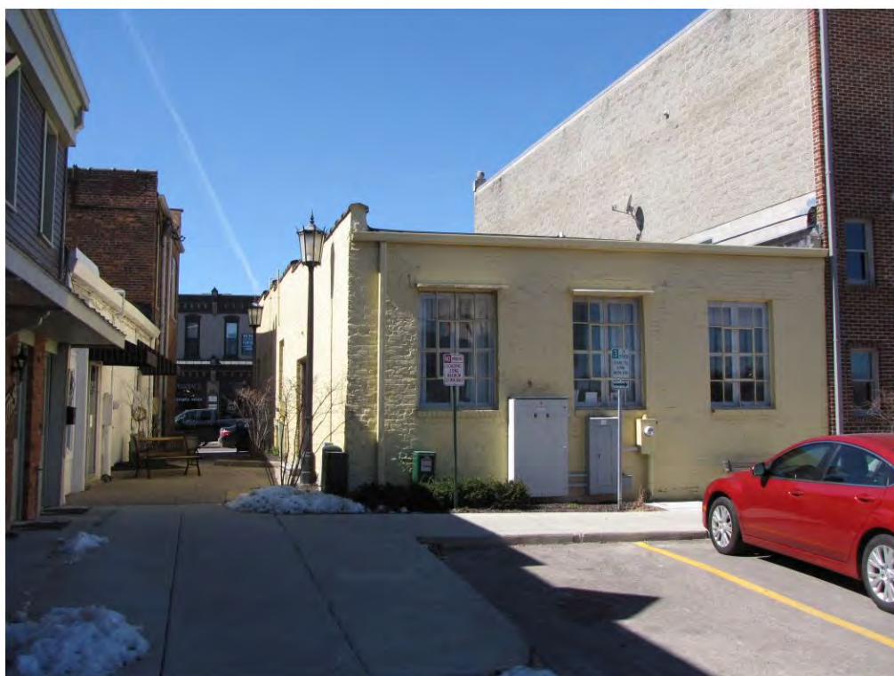
Center North 120_Looking West
