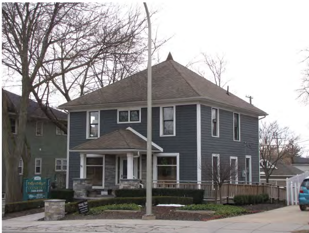
Main East 422_Looking Southeast
