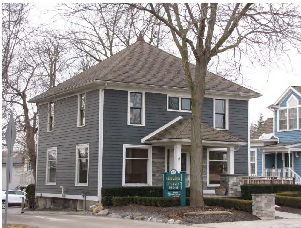
Main East 422_Looking Southwest
