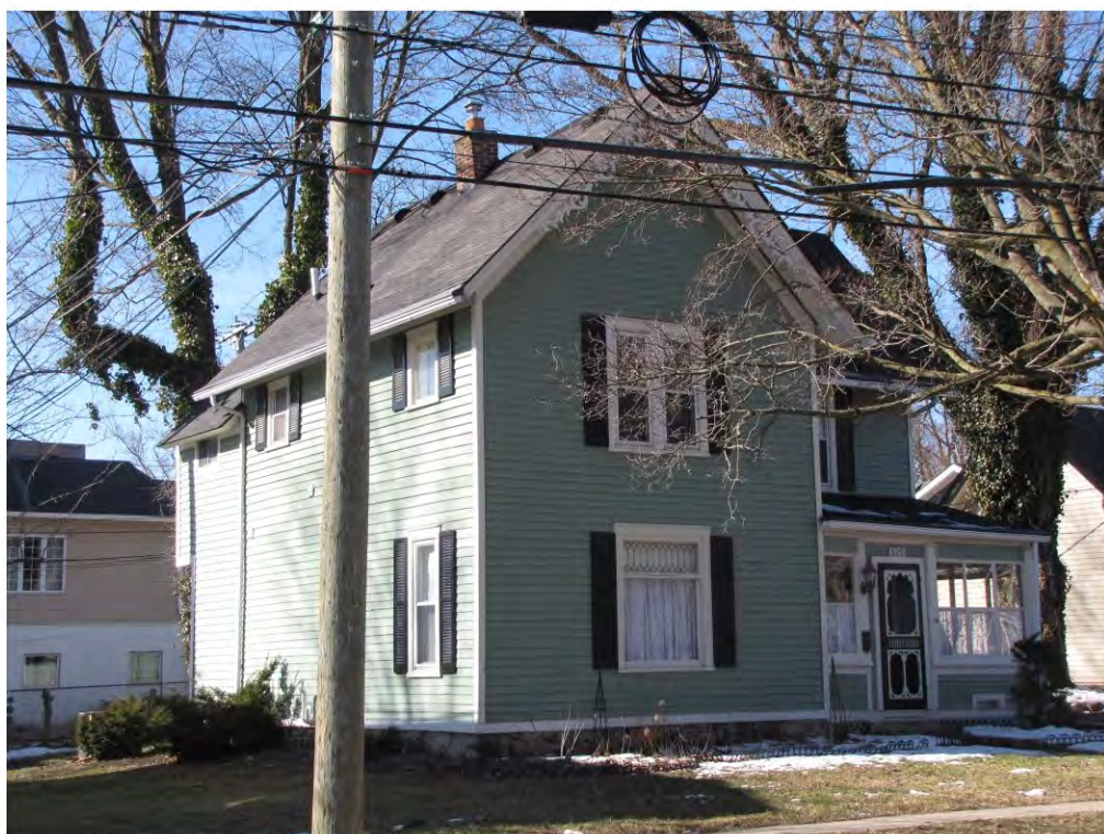
Randolph 125_Looking Southwest
