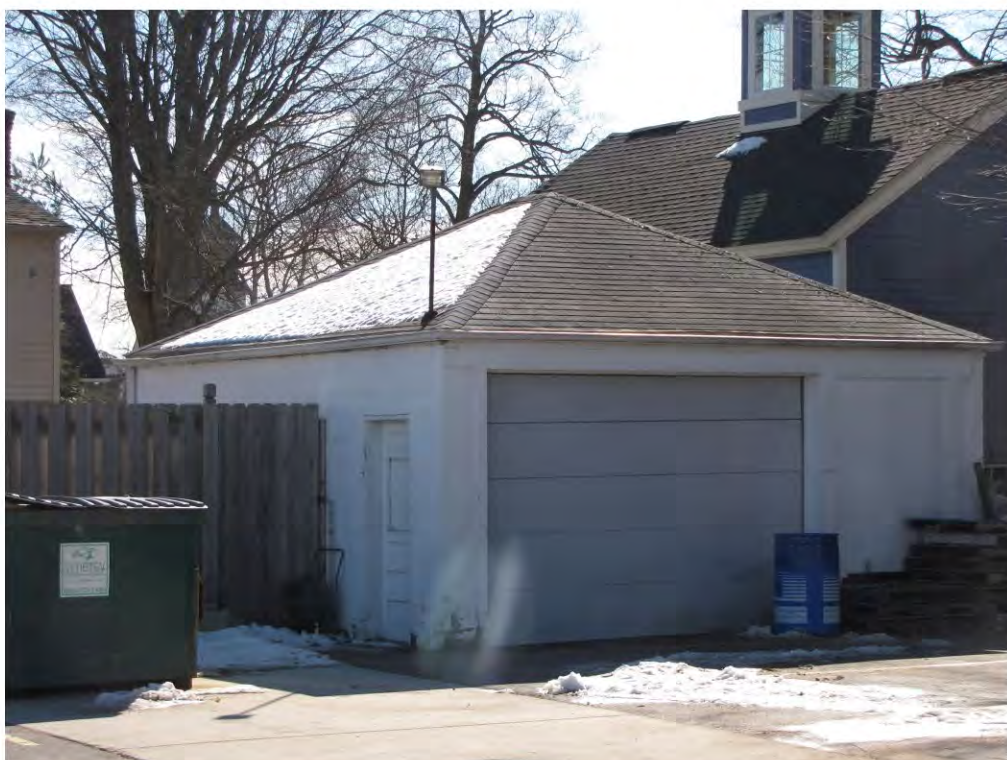
Wing North 217, Garage_Looking Southeast
