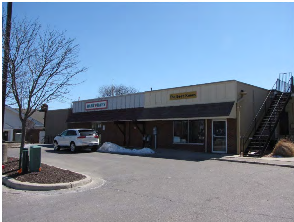
Main East 149_Looking Southwest
