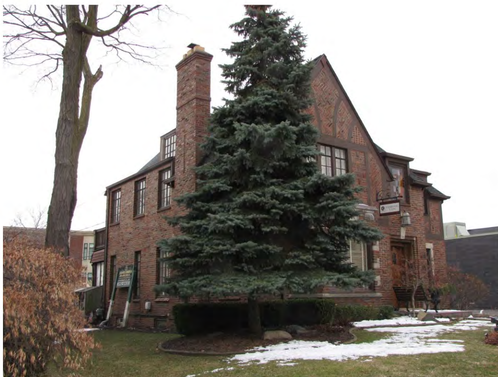
Main East 324_Looking Southwest
