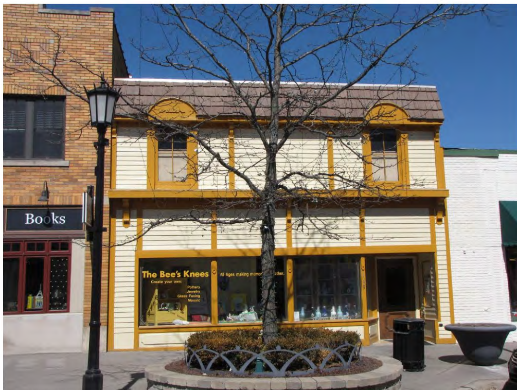
Main East 149_ Looking Northeast
