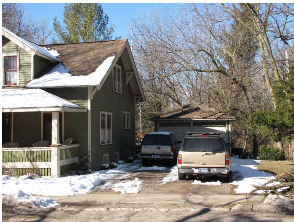
Rogers North 131, Garage_Looking West
