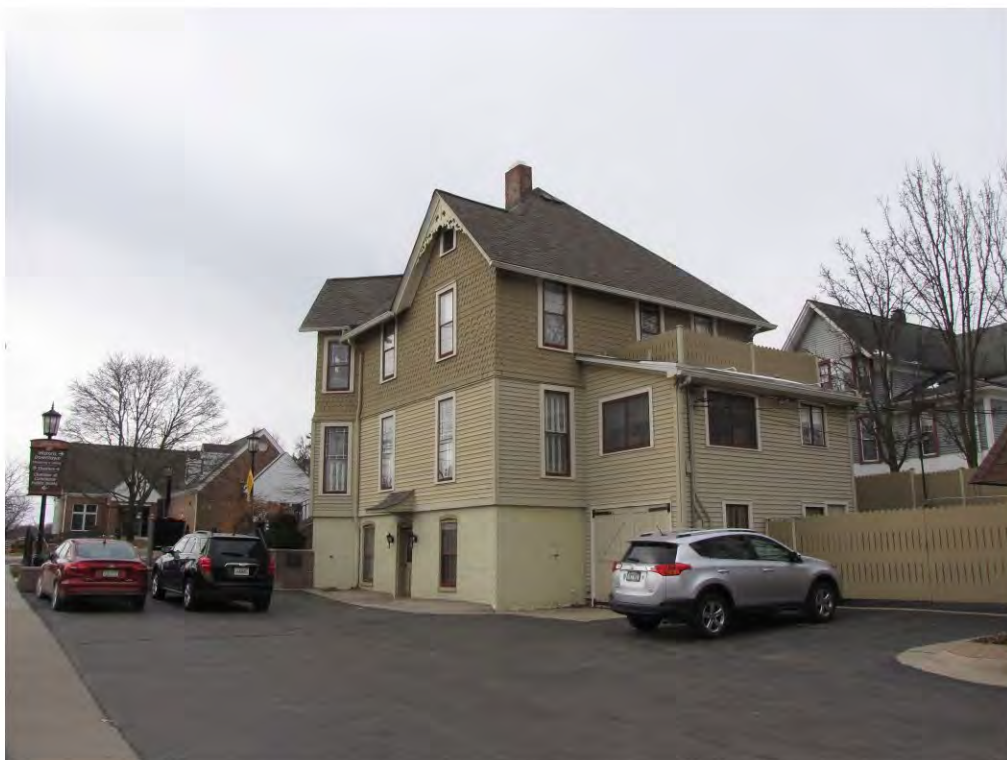
Main East 371_Looking Southwest
