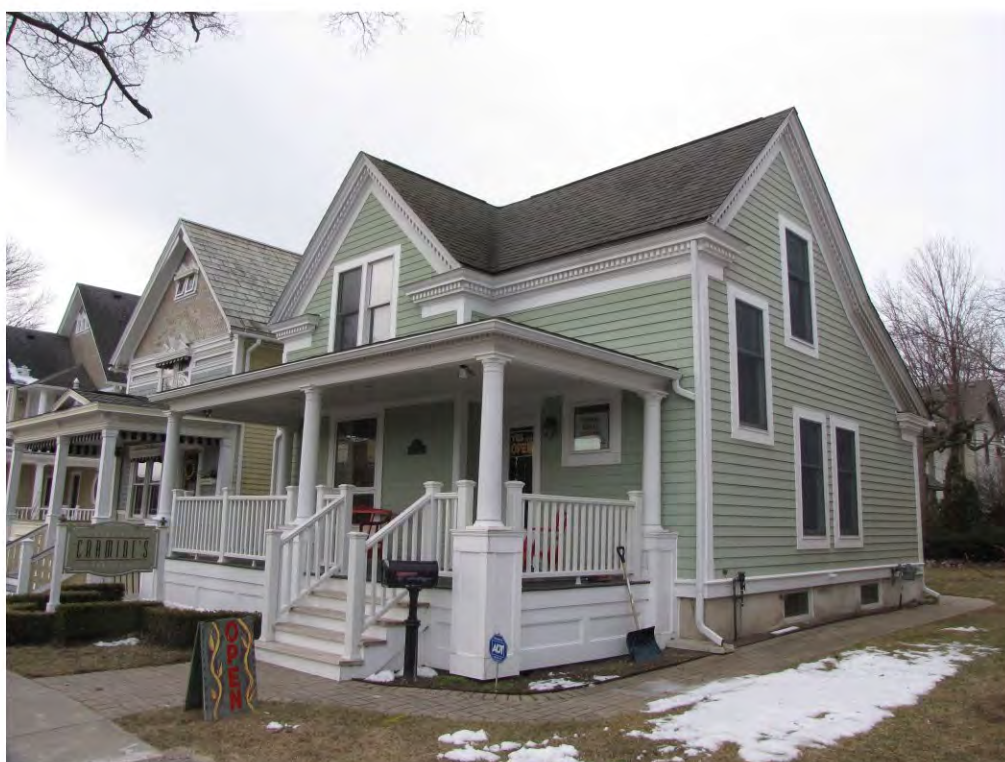
Wing North 125_ Looking Southwest
