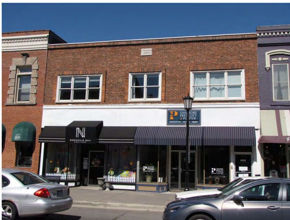
Main East 103-107_Looking Southwest
