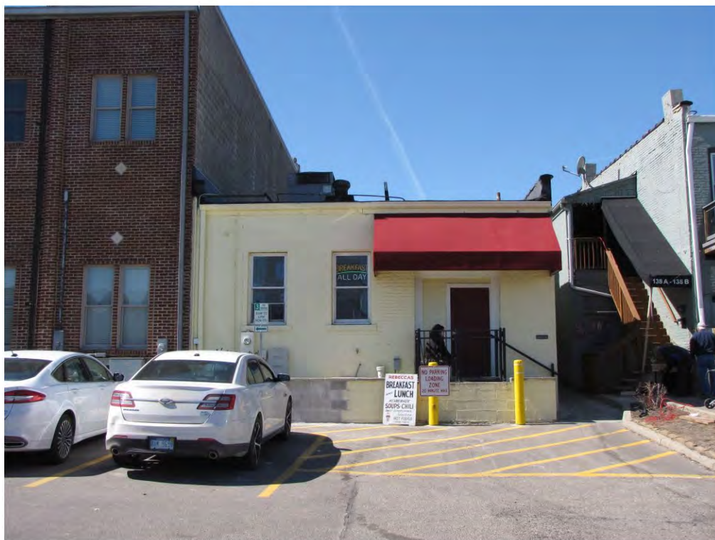
Center North 134_Looking West
