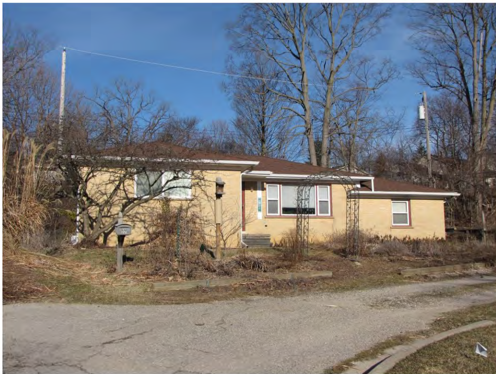
Linden Court 531_ Looking Northwest
