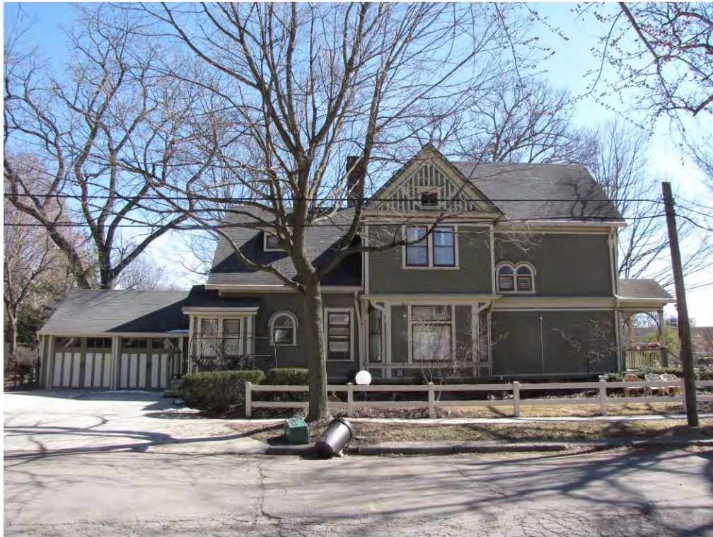
Main West 418_Looking East
