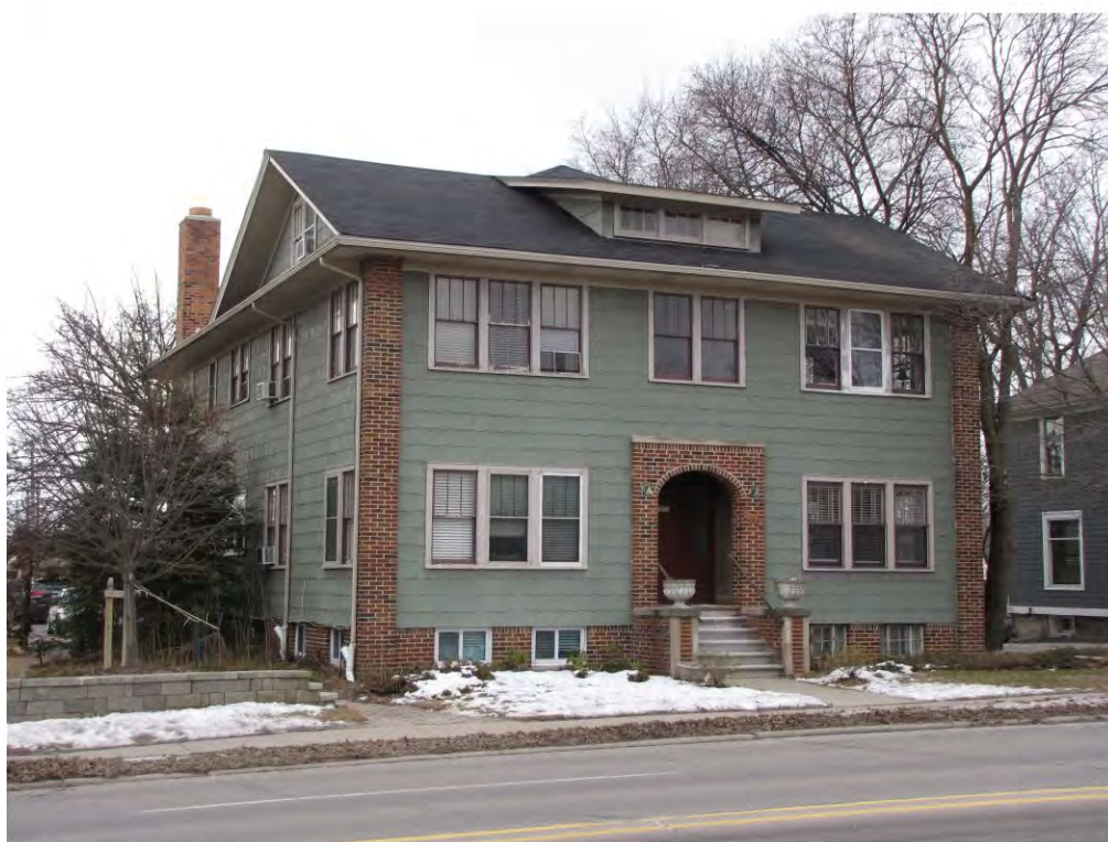
Main East 430_Looking Southwest
