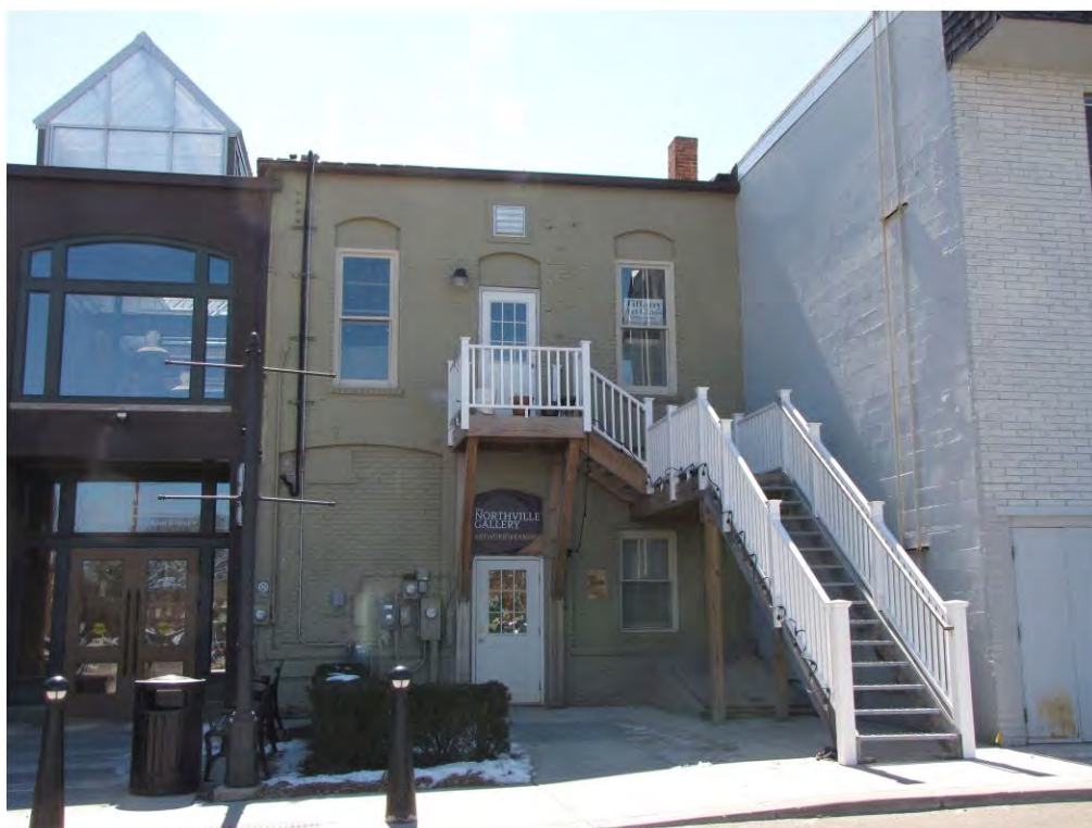
Main East 121-123_Looking South
