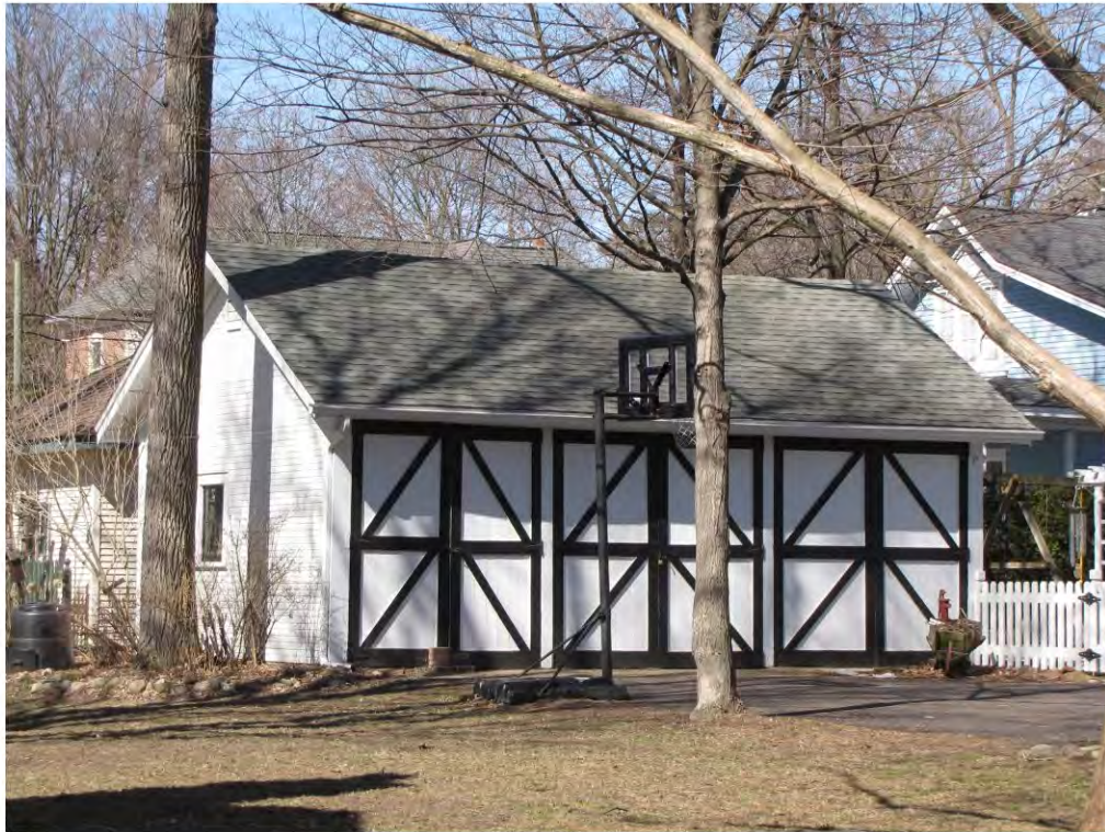
West 121, Garage_Looking Northwest
