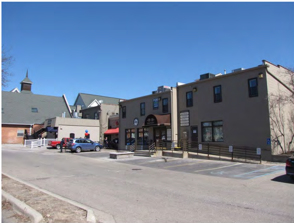
Center North 109-115_Looking Northeast
