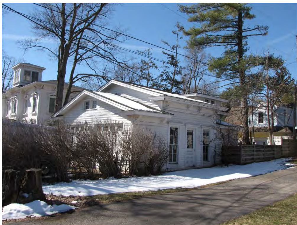
Dunlap West 404, Garage_Looking Southwest
