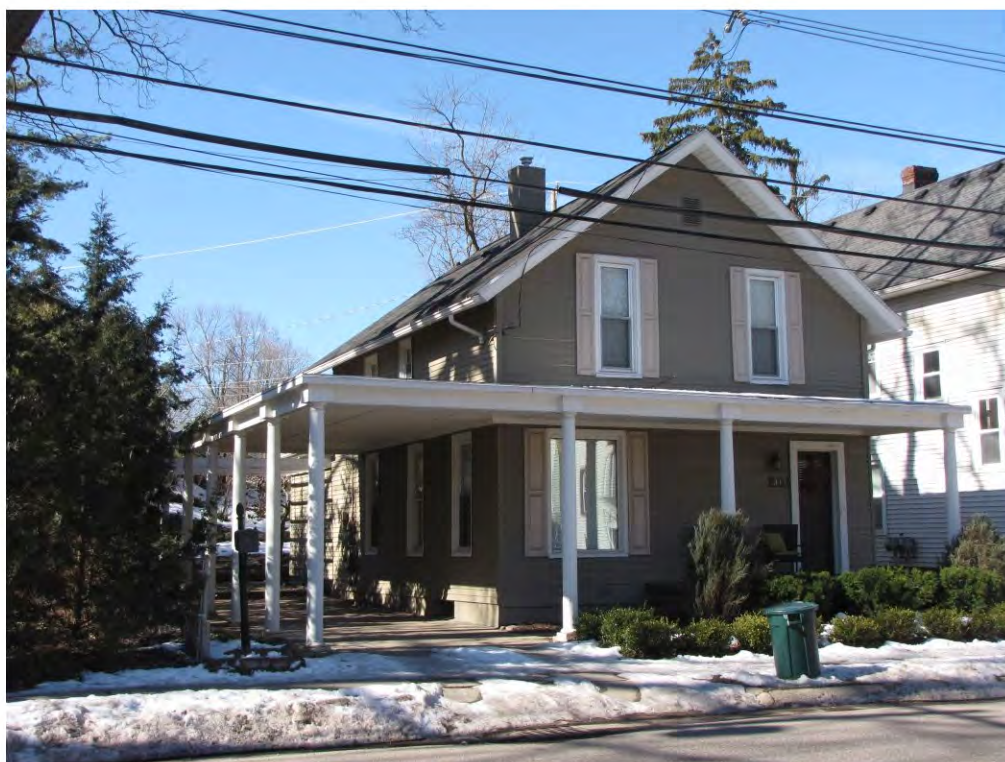
Randolph 317_Looking Southwest
