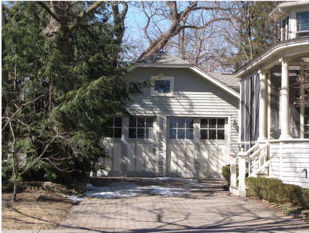
West 113, Garage_Looking West
