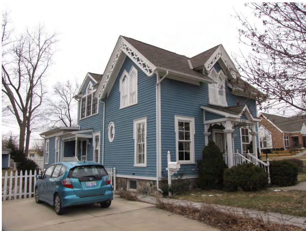
Main East 410_Looking Southwest
