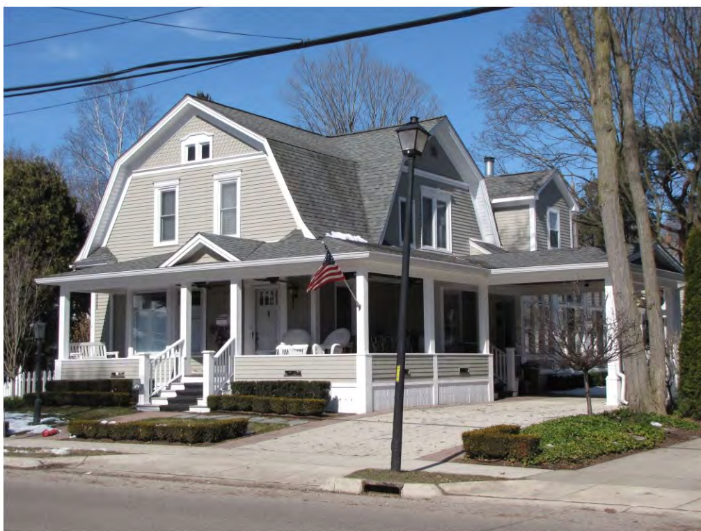
Main West 542_Looking Northwest
