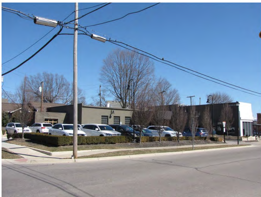
Main West 202_Looking Northeast
