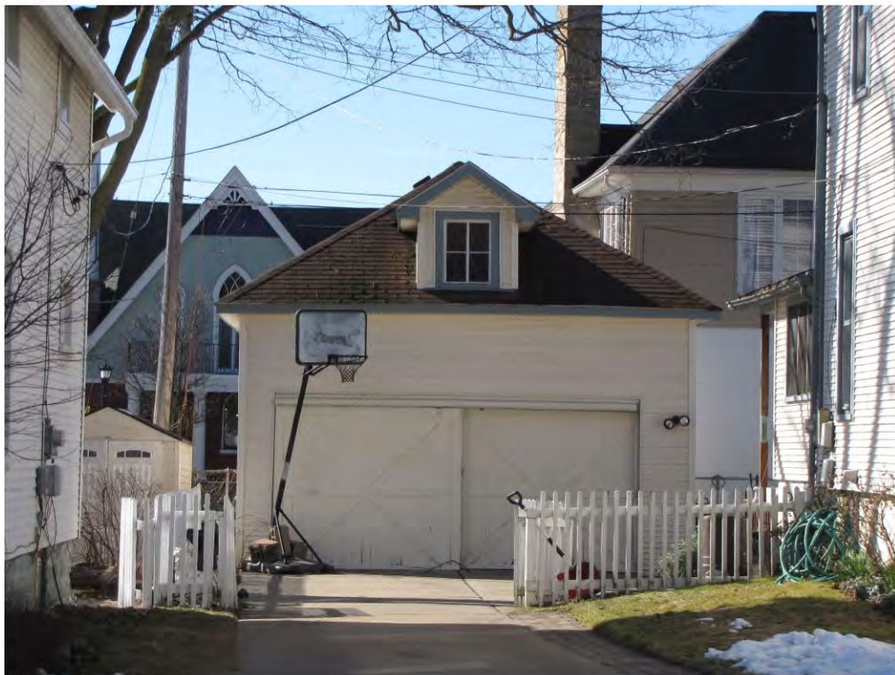
Randolph 119, Garage_Looking South
