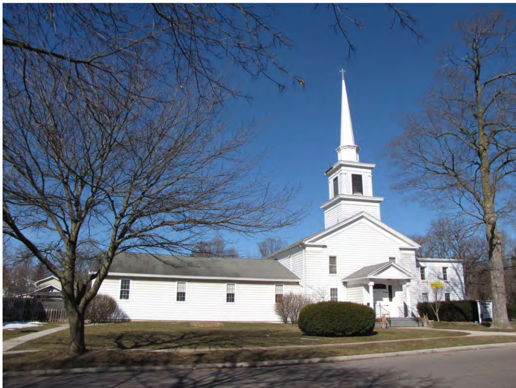
Wing North 217_Looking Northwest
