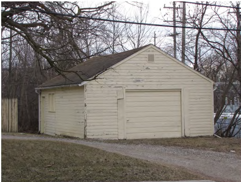
Cady East 350, Garage_Looking Southeast
