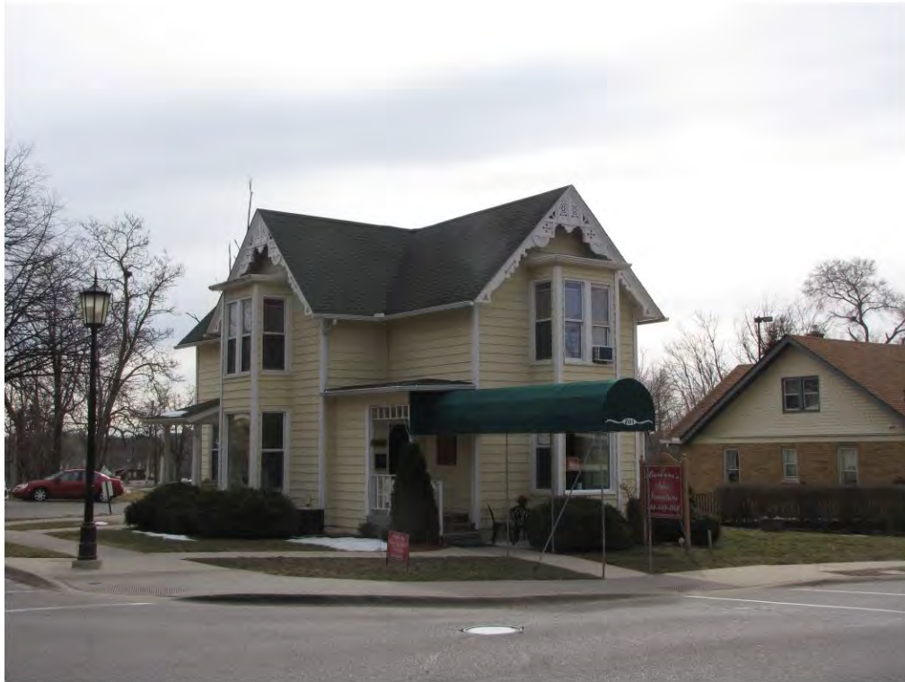
Center South 201 and Cady East 100_Looking Southeast
