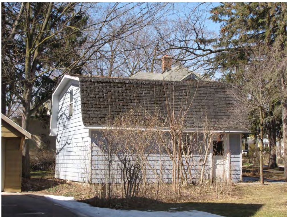
Dunlap West 305, Garage_Looking West
