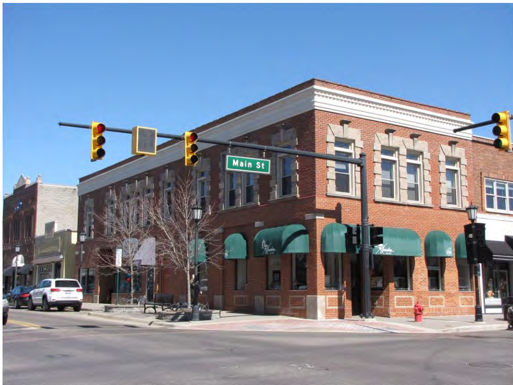
Main East 101 and Center North 108-110_Looking Northeast
