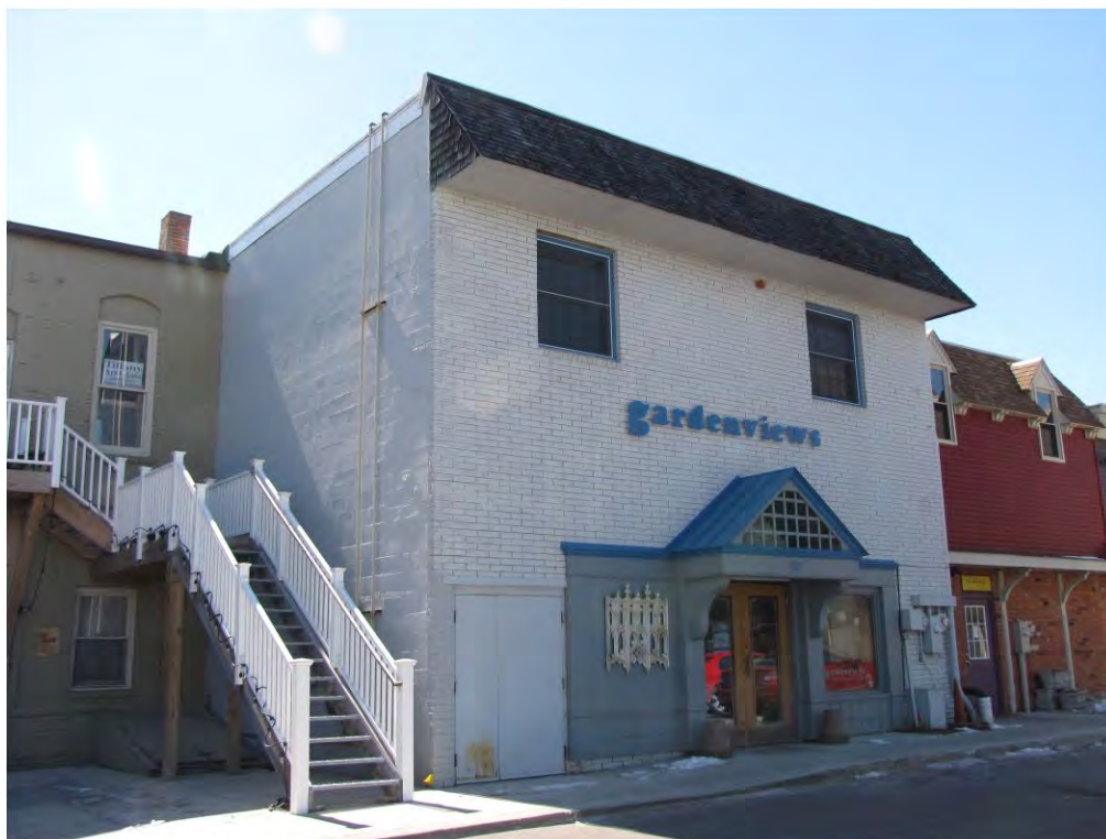
Main East 117_Looking Southwest
