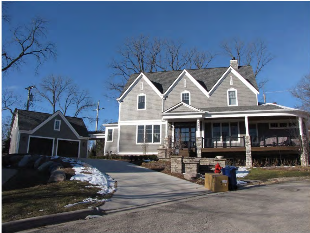
Linden Court 525_Looking Southwest
