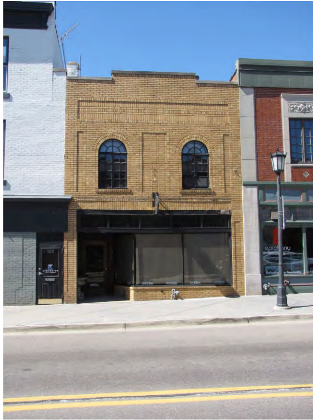
Center North 105_Looking West
