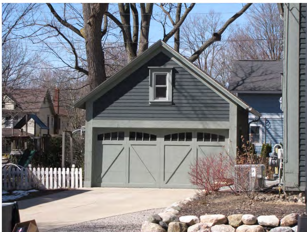
Dunlap West 401, Garage_Looking West
