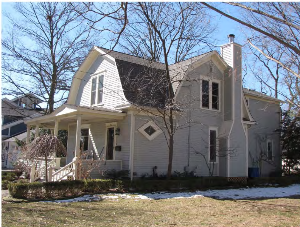
West 113_Looking Southwest
