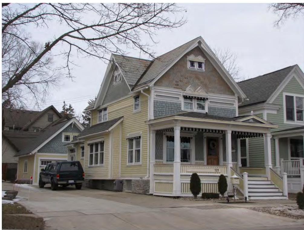
Wing North 121_Looking Northwest
