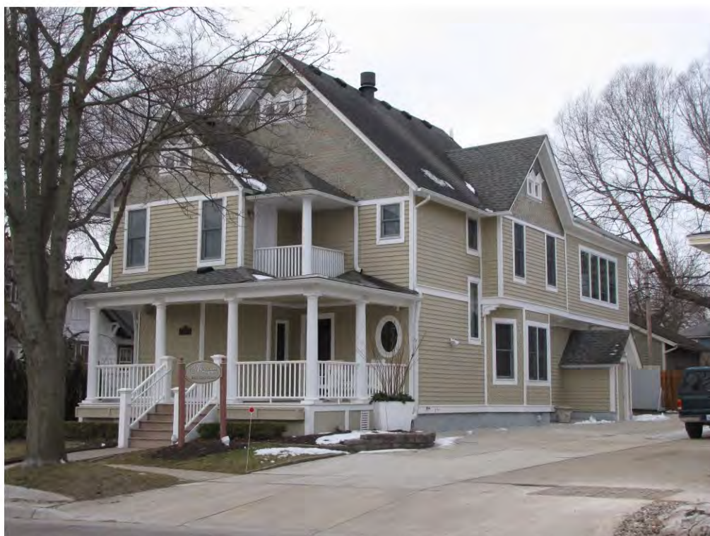
Wing North 117_Looking Southwest
