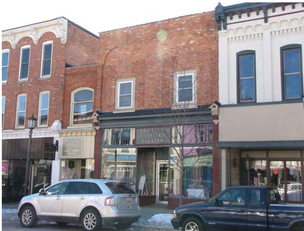
Main East 112_Looking Southeast
