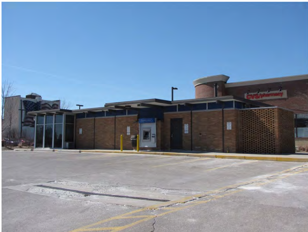
Dunlap East 143_Looking Southwest
