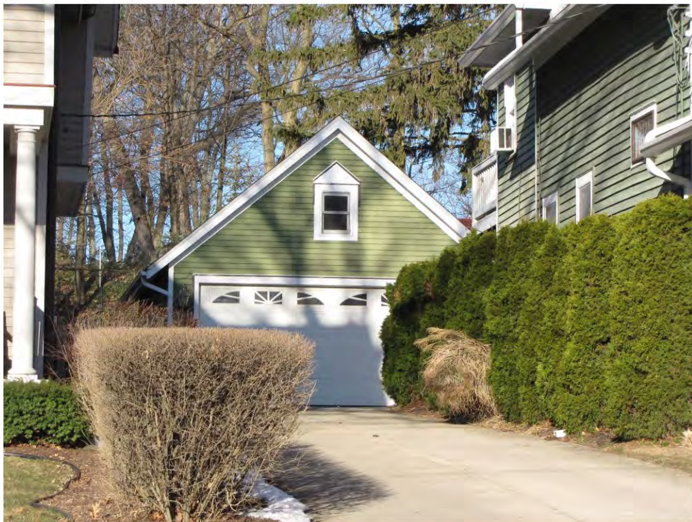
Rogers North 359, Garage_Looking West
