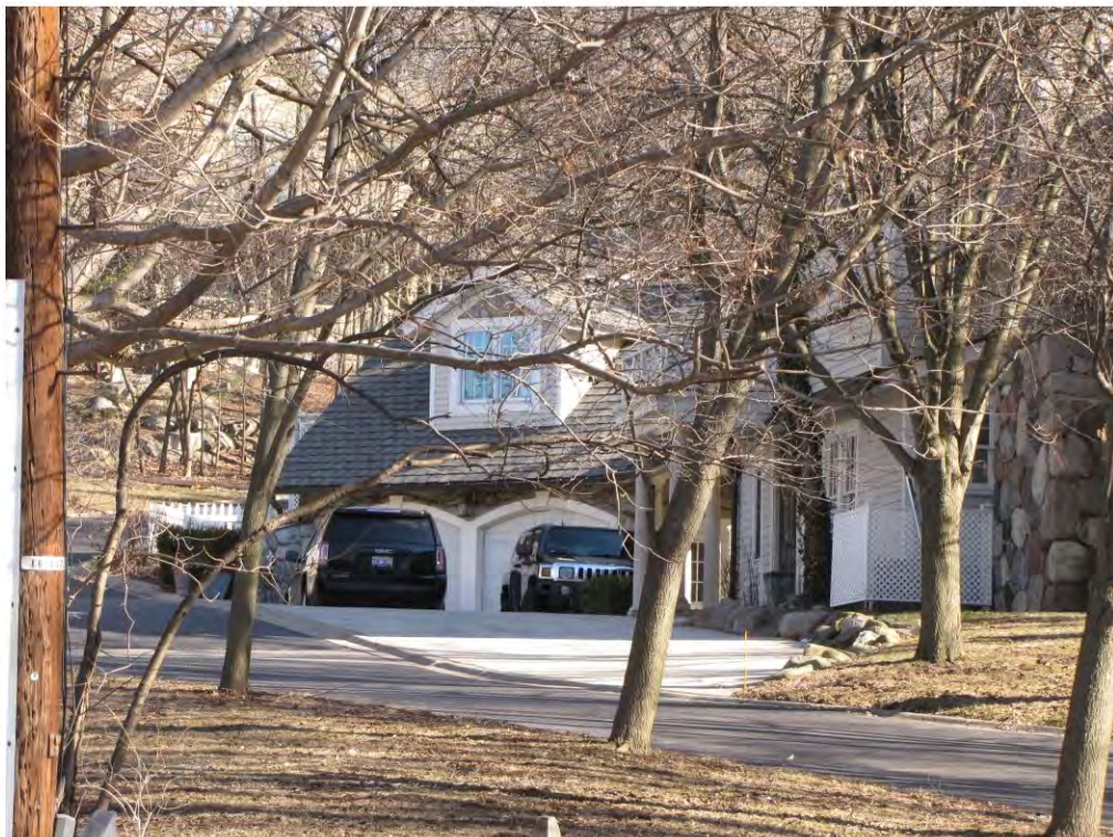
Randolph 562, Garage_Looking North
