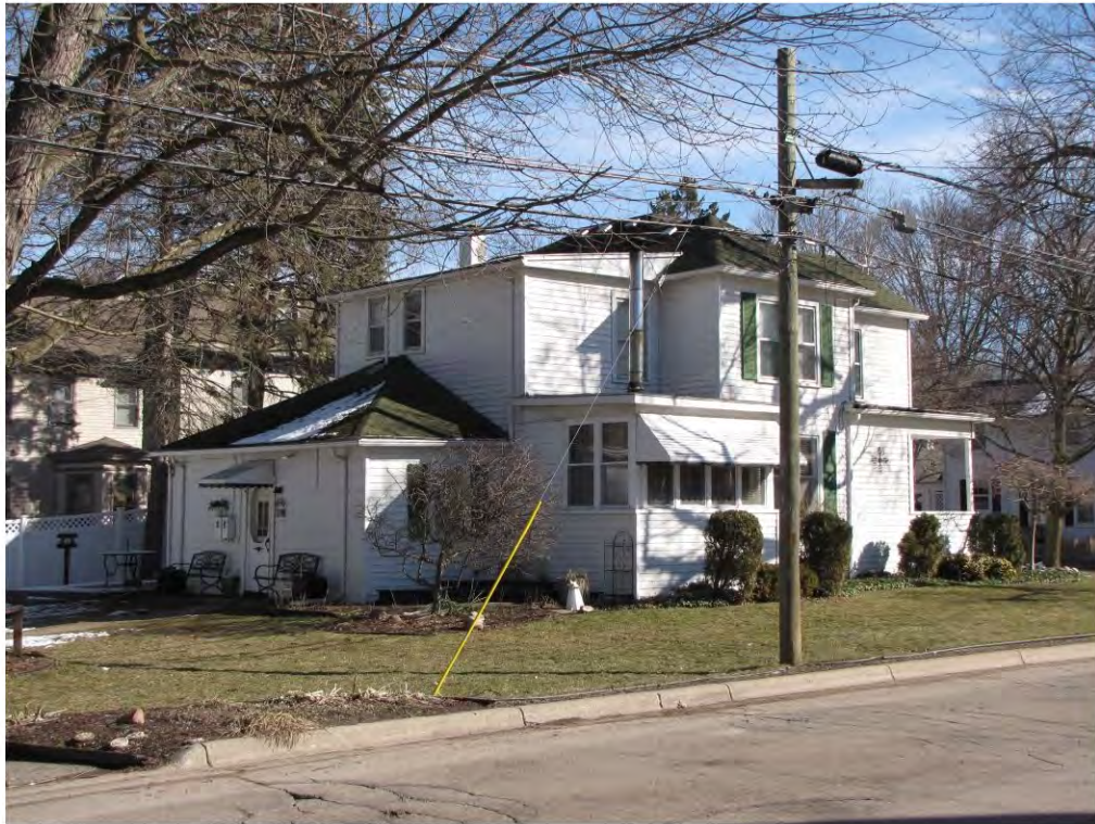
Rogers North 101_Looking Northeast
