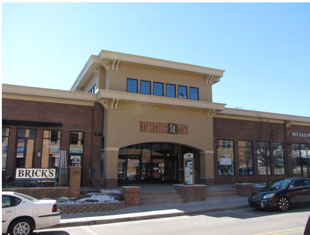
Main West 133_Looking South
