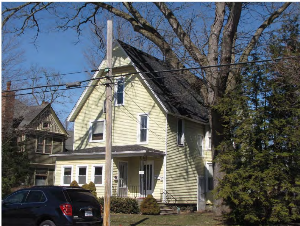
Main West 410_Looking Northwest
