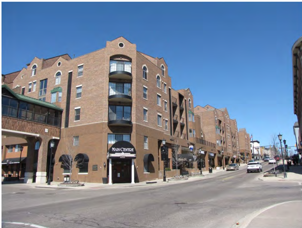
MainCentre 150_Looking Northwest
