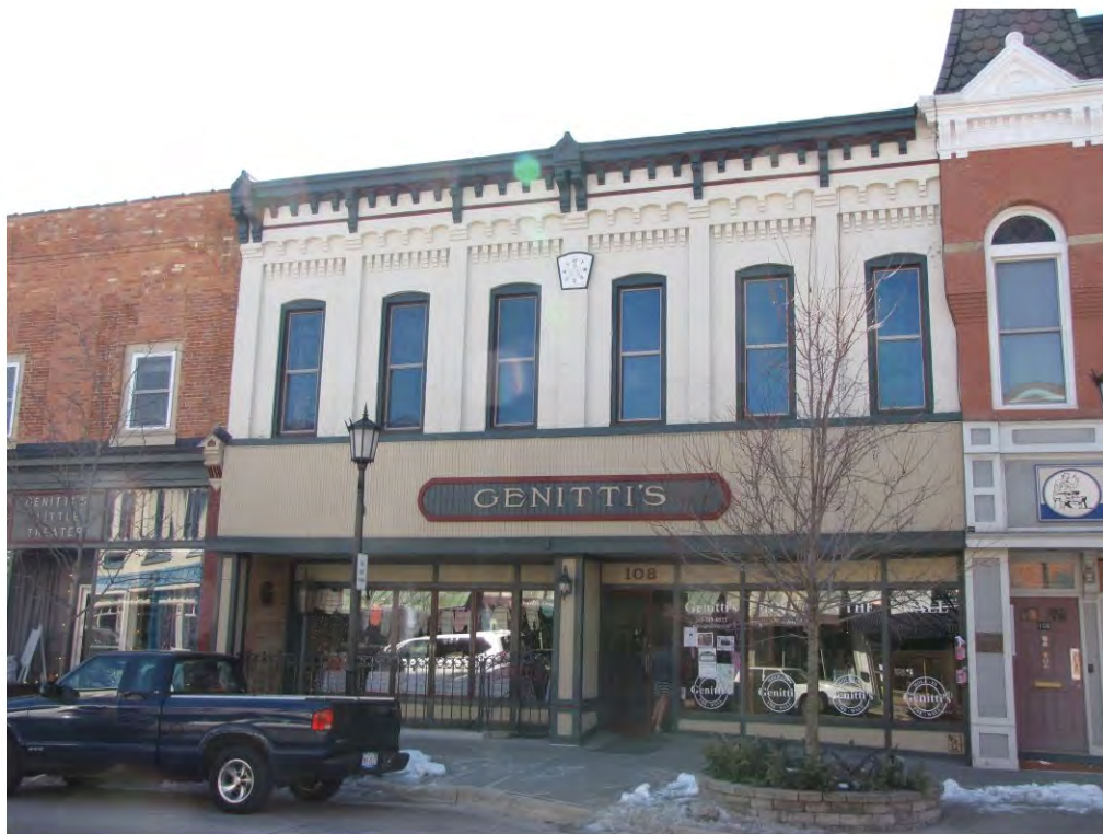
Main East 108-110_Looking Southwest
