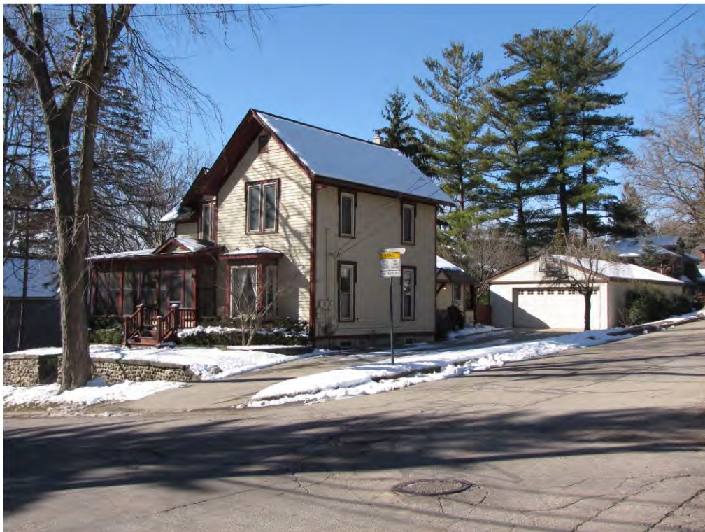
Rogers North 231, Garage_Looking West
