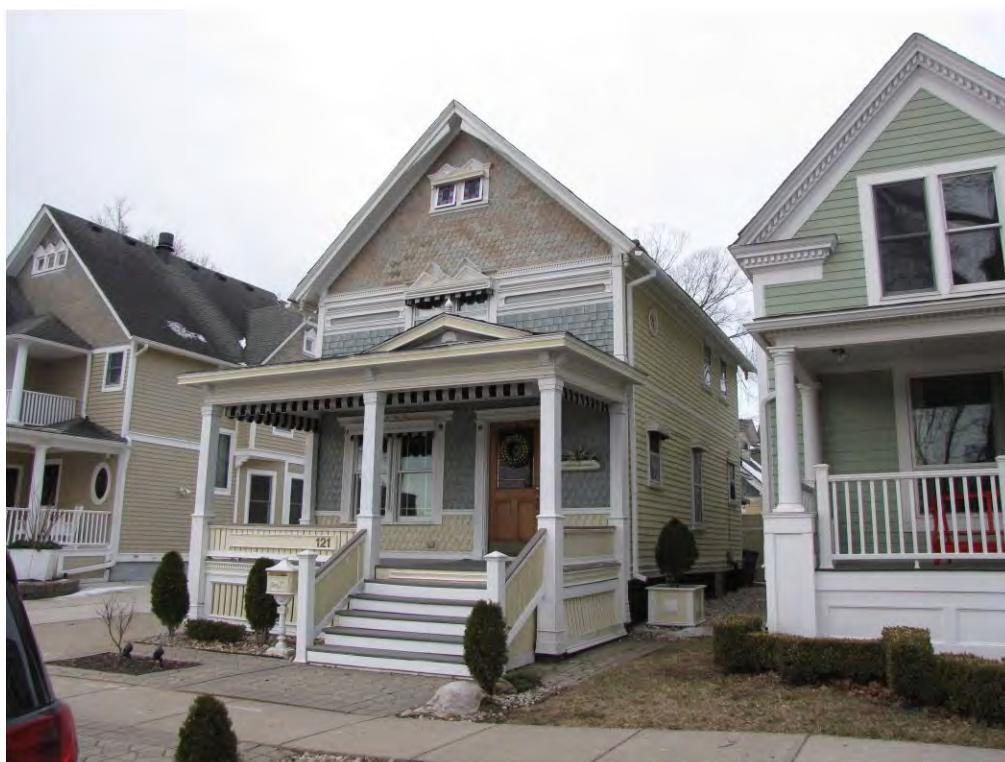
Wing North 121_Looking Southwest
