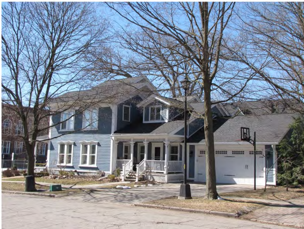
Main West 404_Looking Southwest
