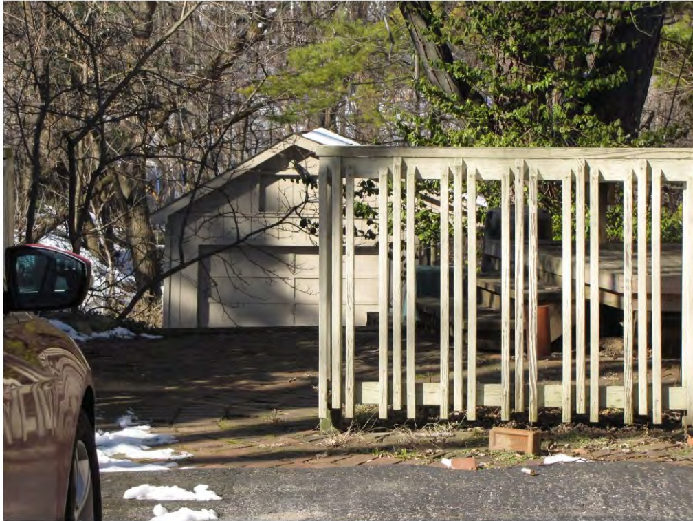
Randolph North 117, Garage_Looking West
