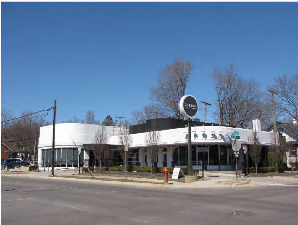
Main West 202_Looking Northwest
