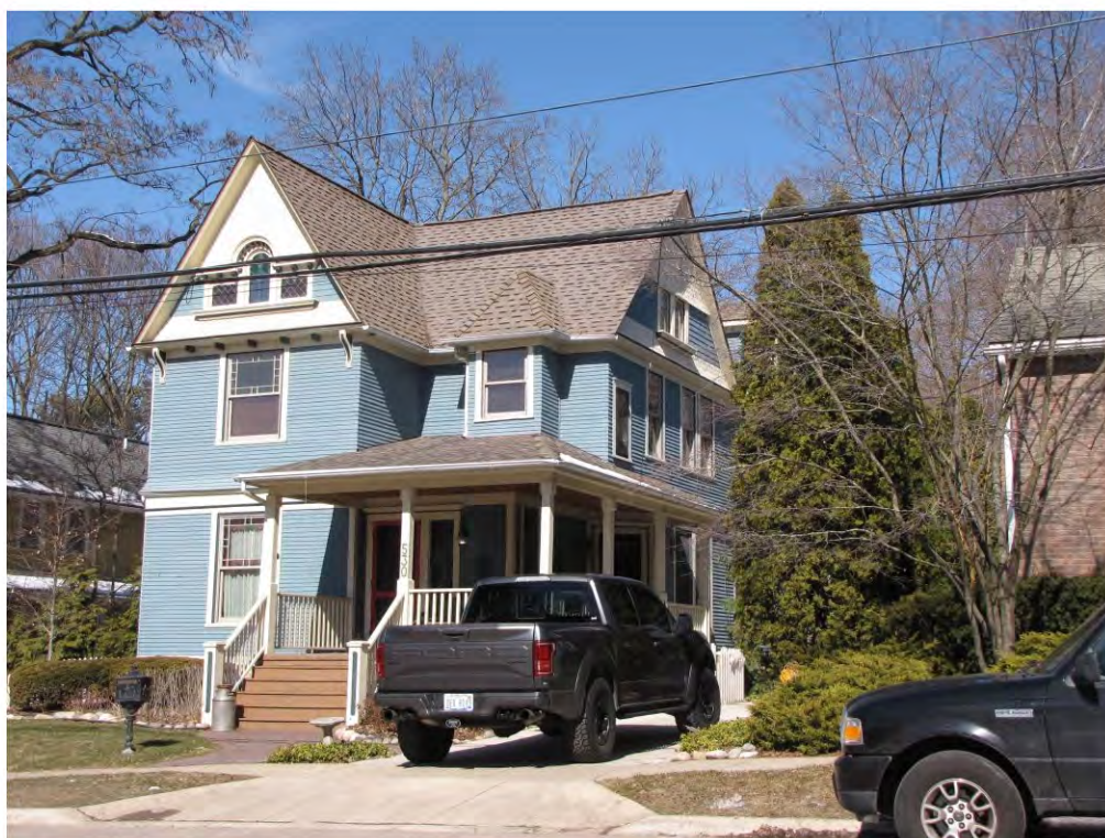
Main West 530_Looking Northwest
