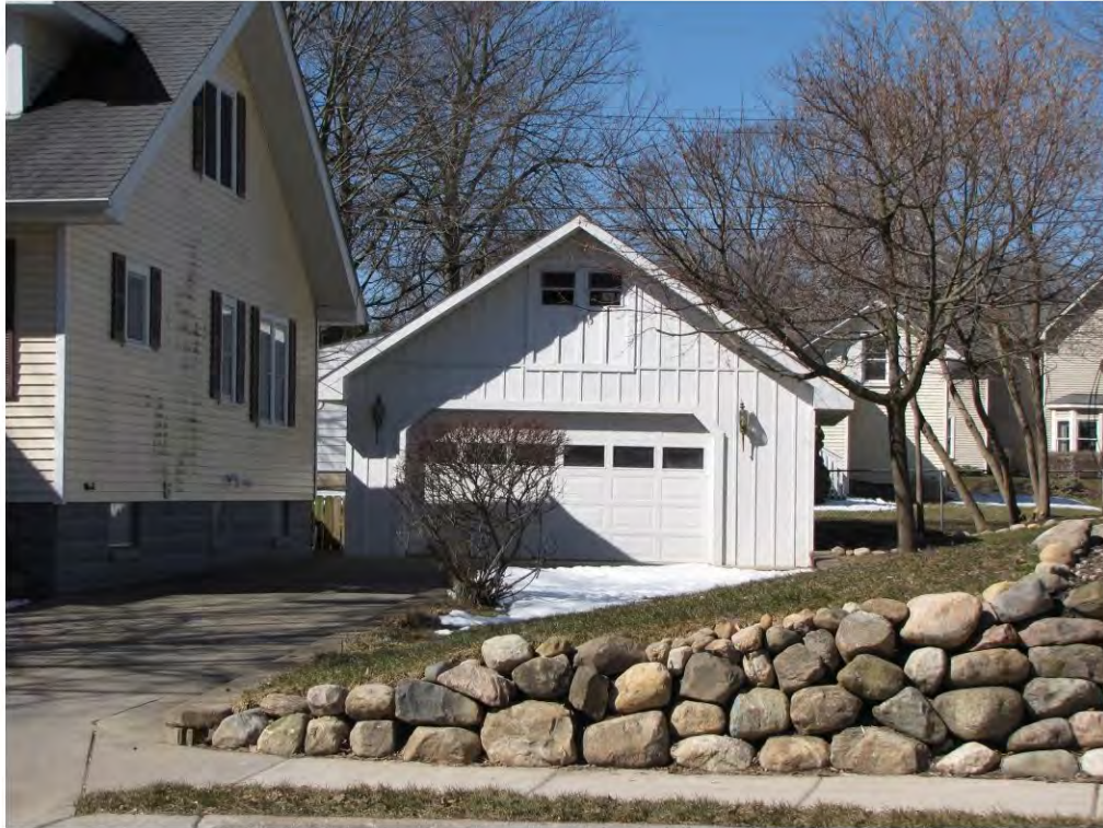
West 231, Garage_Looking West
