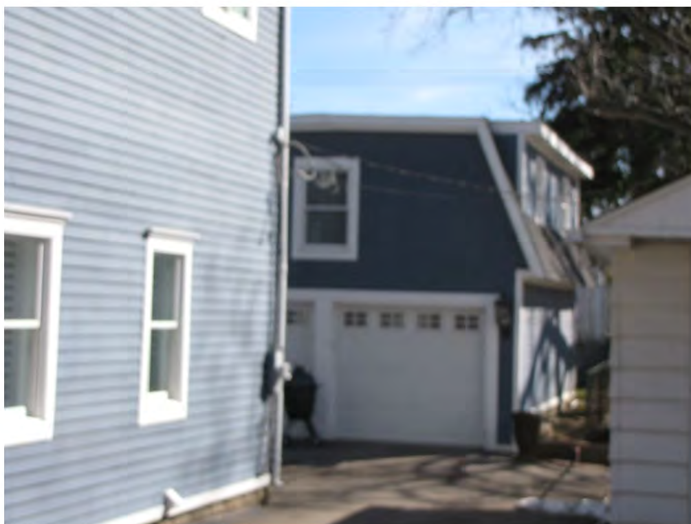
Linden 254, Garage_Looking East
