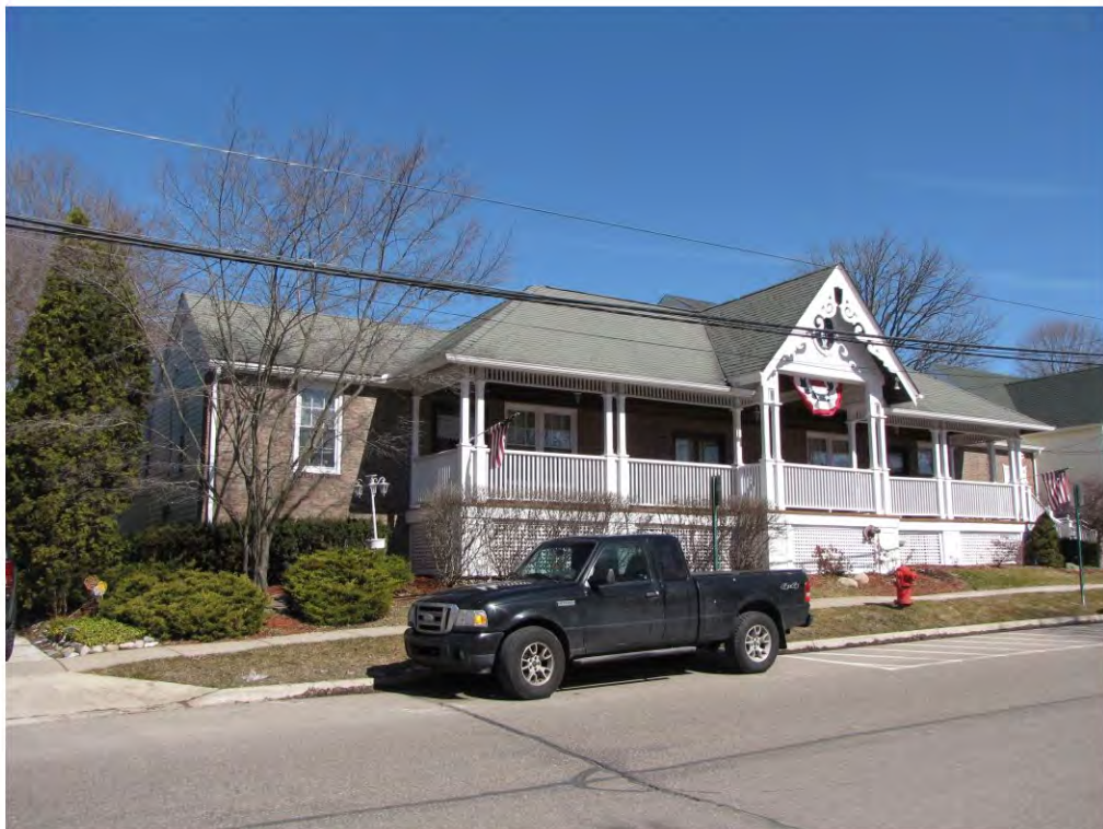
Main West 520_Looking Northeast
