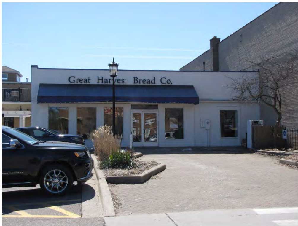
Main East 139_Looking South
