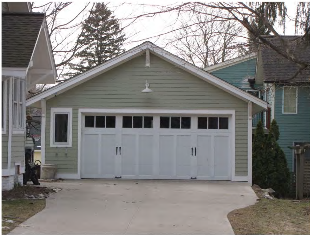
Cady West 487, Garage_Looking South
