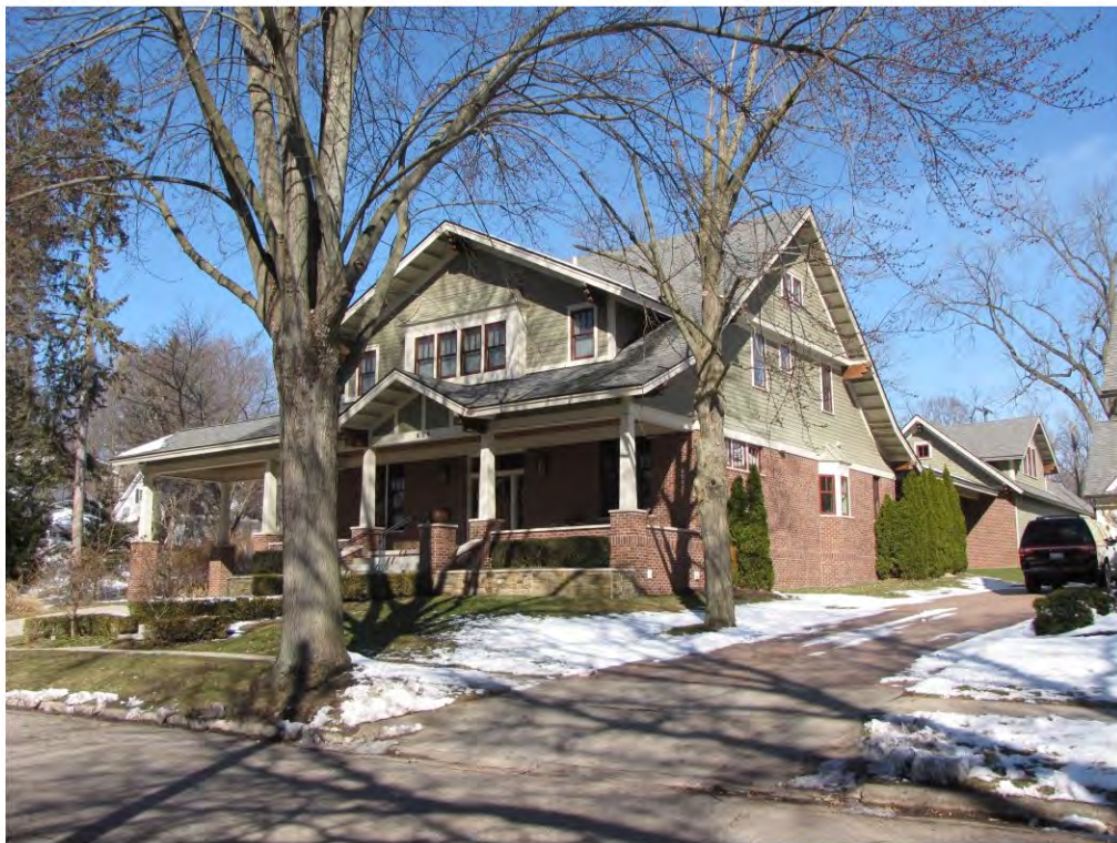
Dubuar 430_ Looking Northwest
