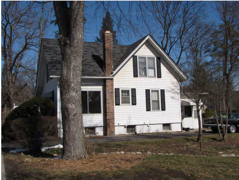
Rogers South 117_Looking Northeast
