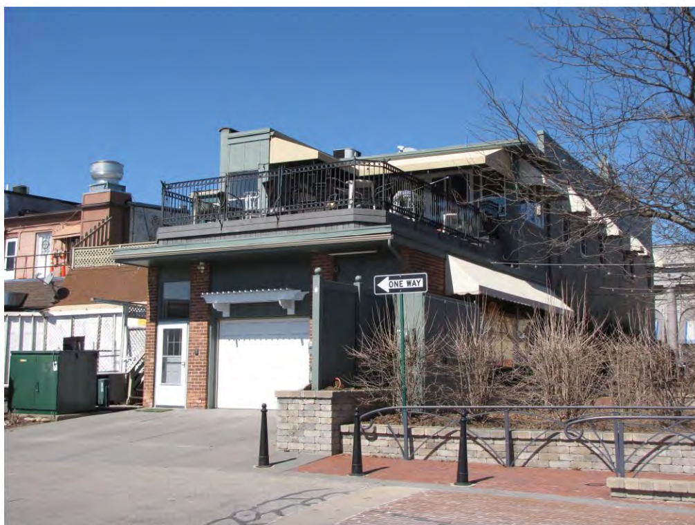
Main East 126-134_Looking South
