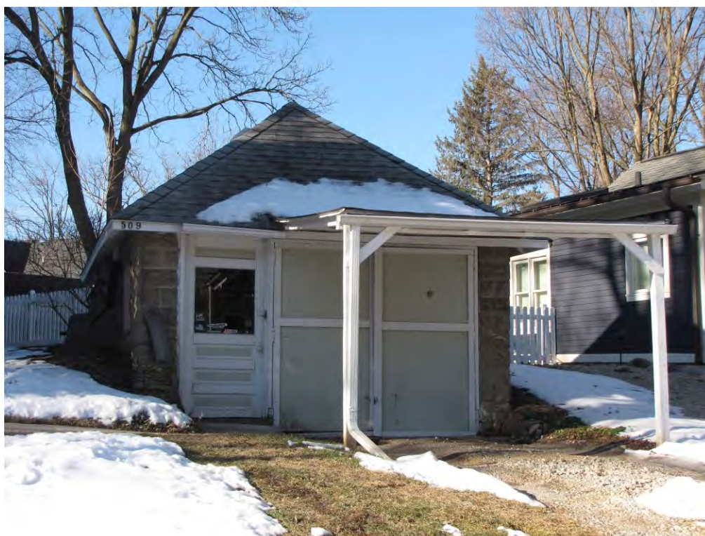
Randolph 509, Garage_Looking South
