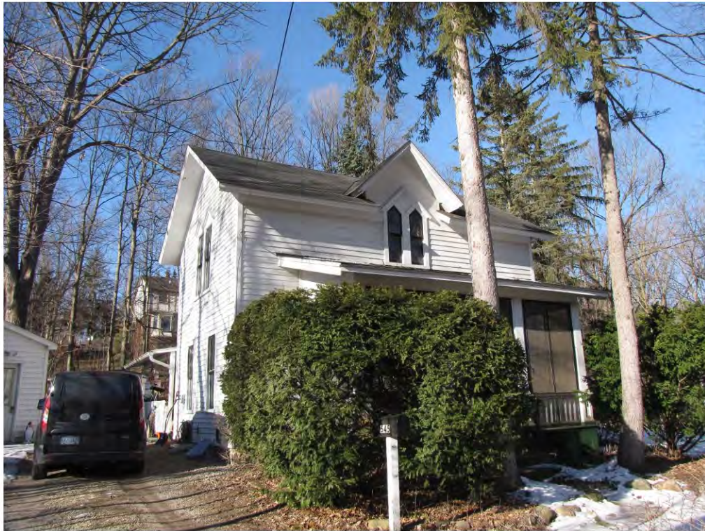
Randolph 545_Looking Southwest
