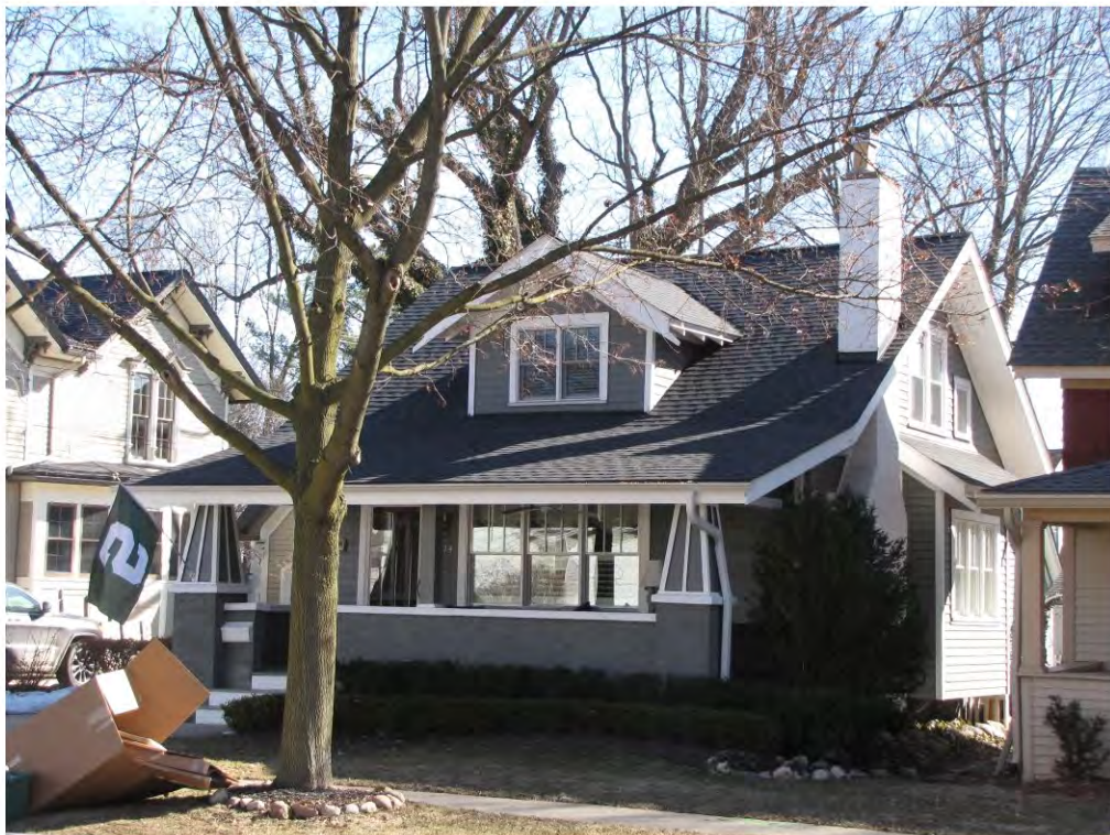
Wing North 214_Looking Northwest
