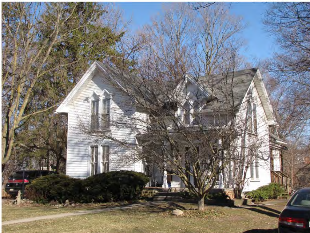
Randolph 132_ looking Northwest
