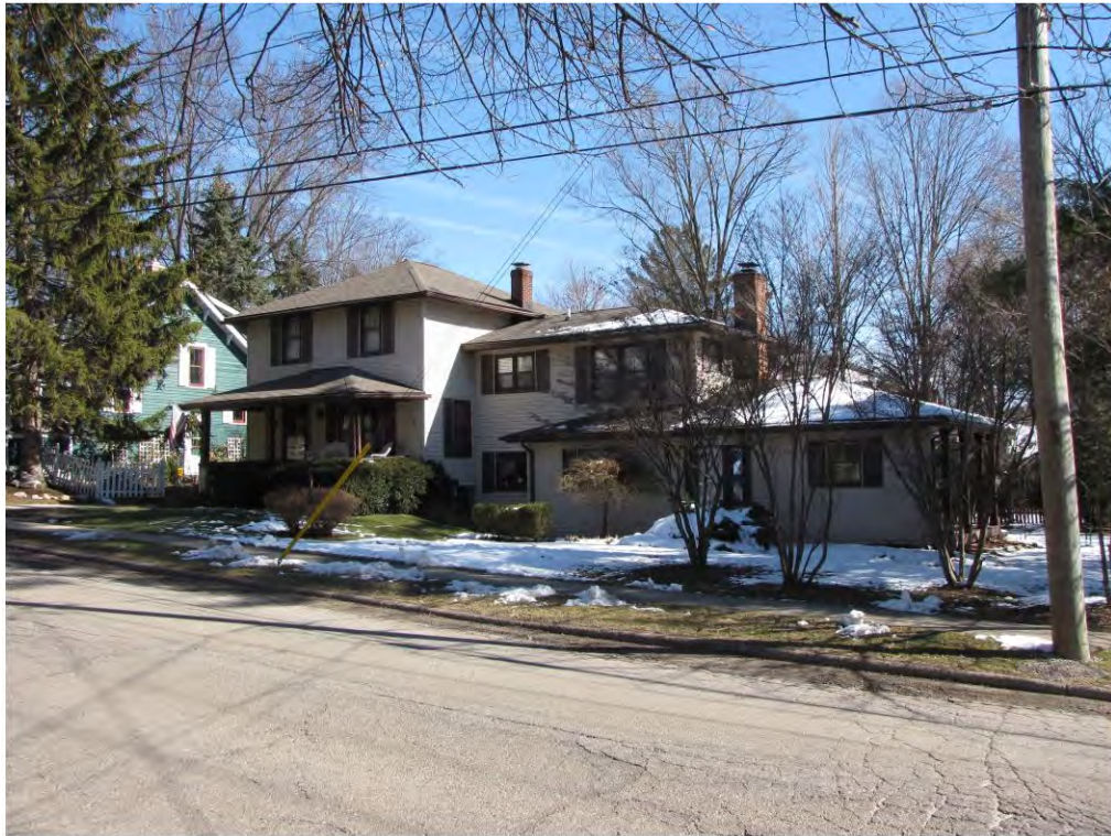
Rogers North 230_Looking Northeast
