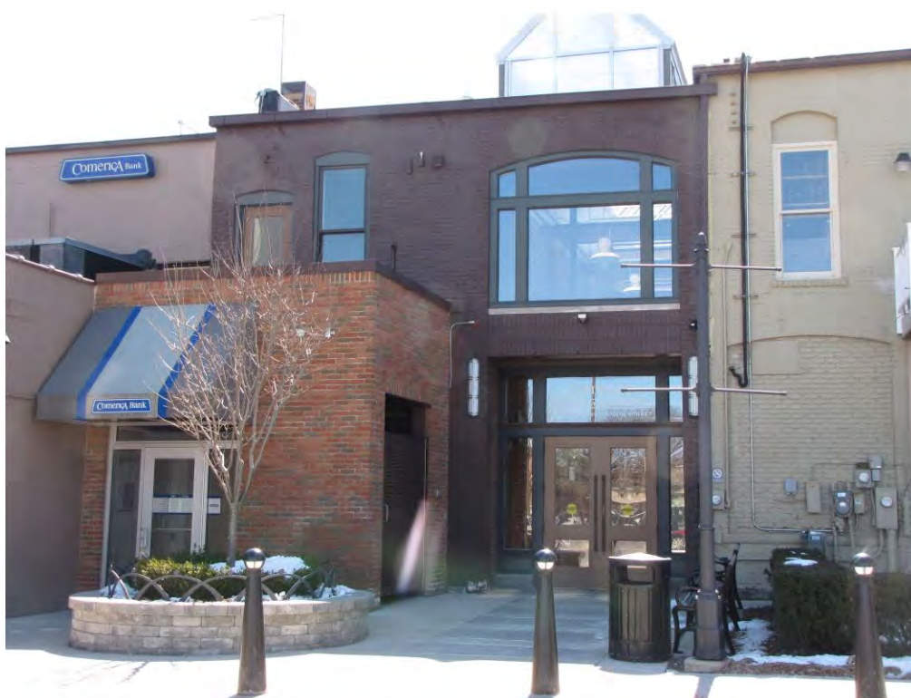
Main East 125_Looking South
