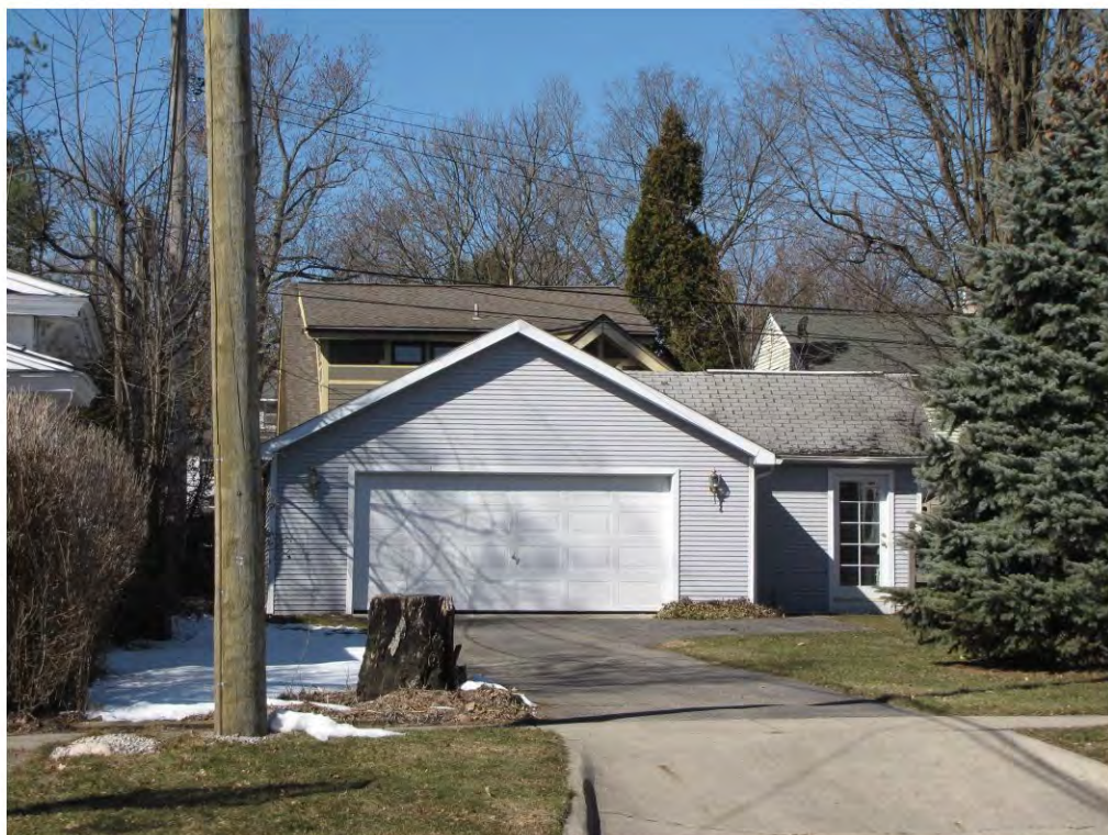
West 223, Garage_Looking West
