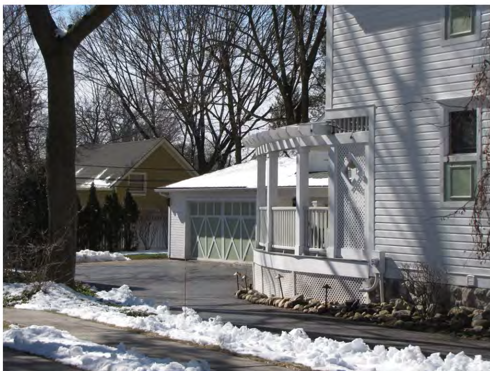
Dunlap West 537, Garage_Looking Southwest
