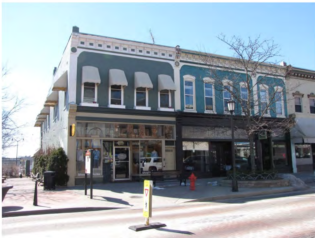
Main East 126-124_Looking Southwest
