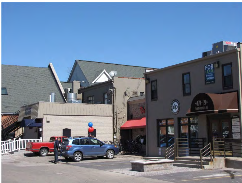
Center North 135-137_Looking Northeast
