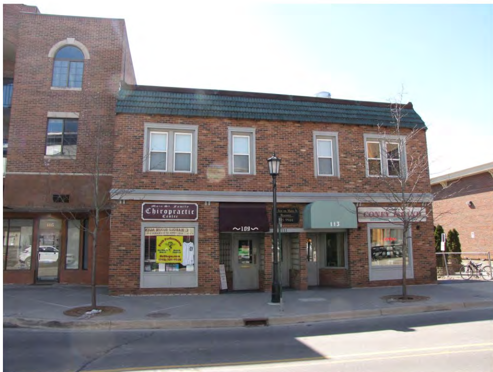
Main West 109-113_Looking South
