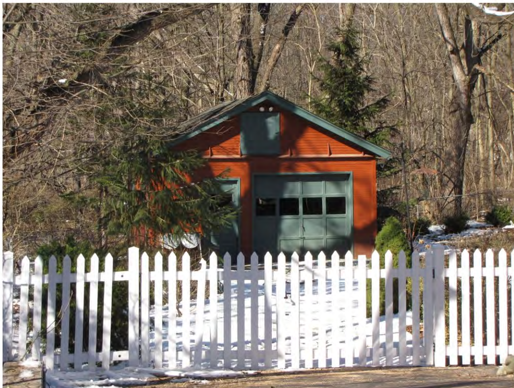
Rogers North 201, Garage_Looking West
