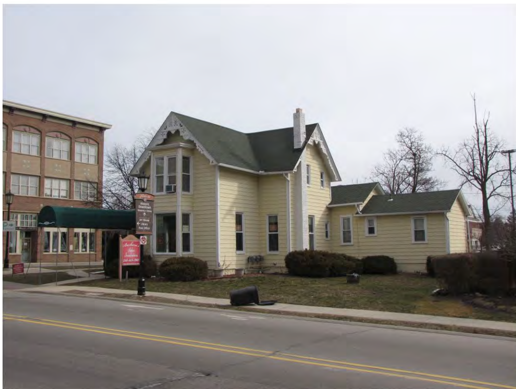
Center South 201 and Cady East 100_Looking Northeast
