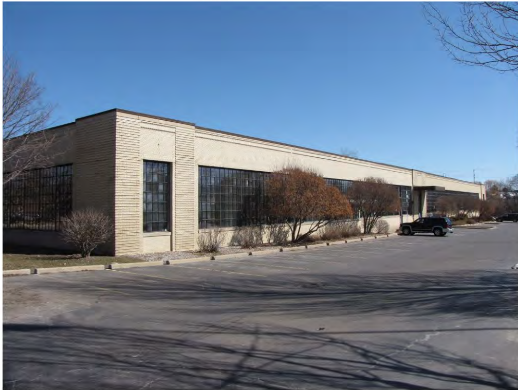
Main East 235_Looking Northeast
