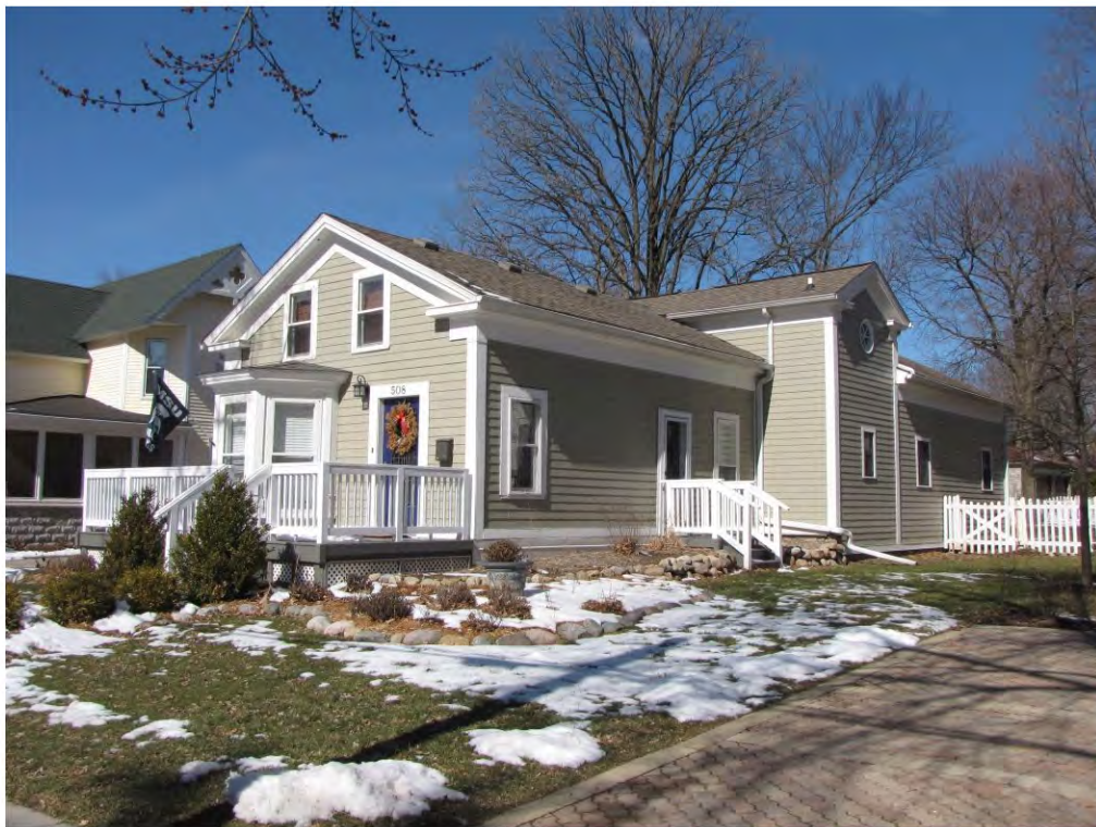
Main West 508_Looking Northwest
