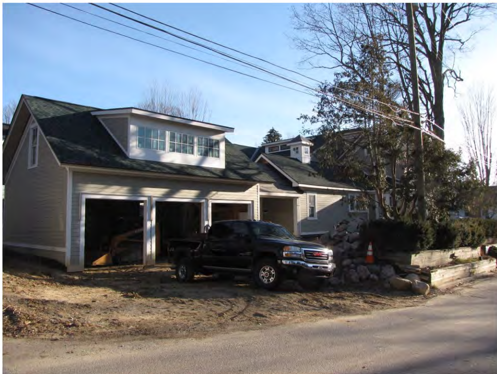
Rogers North 333_Looking Northeast
