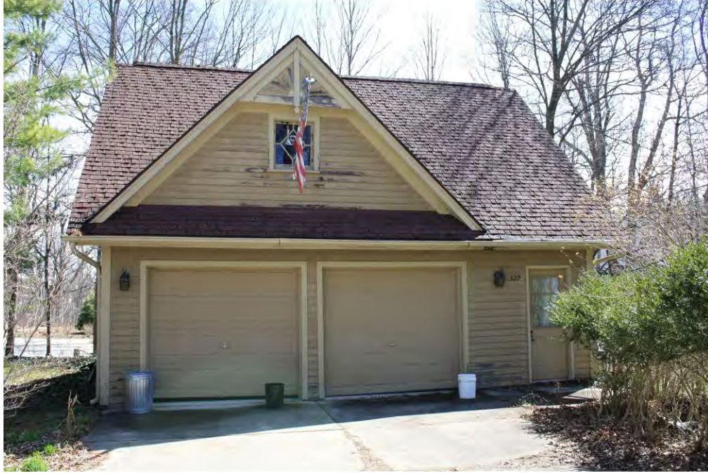
High 320, Garage_Looking East
