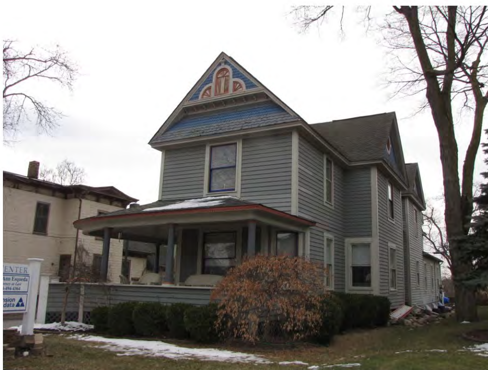
Main East 332_Looking Southeast
