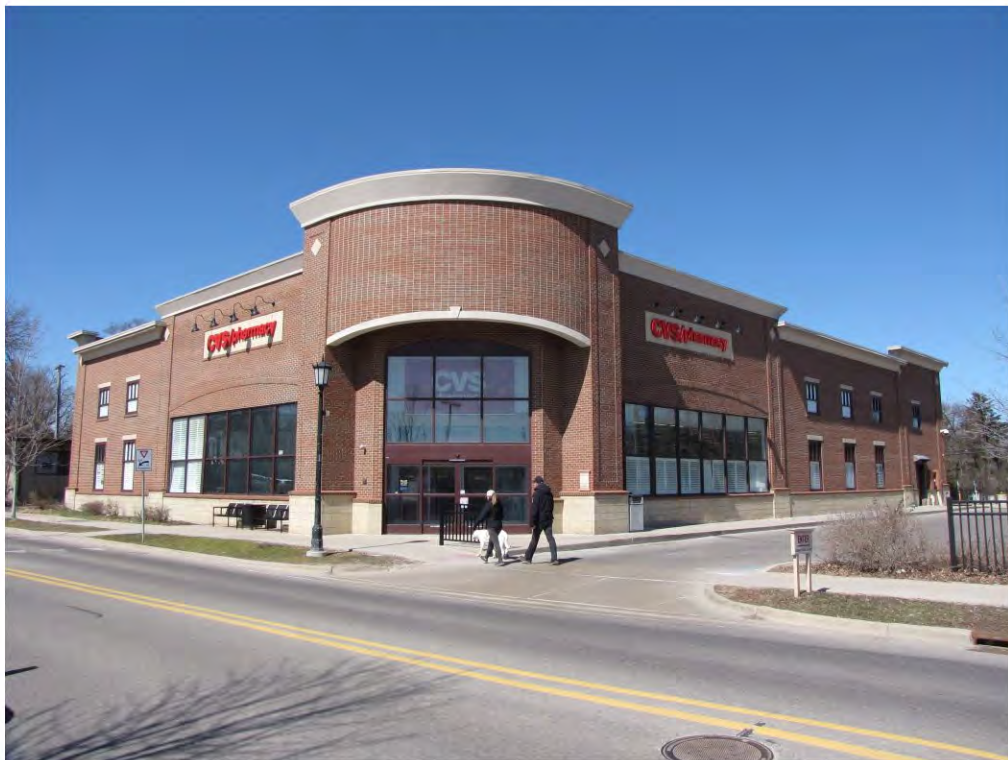
Dunlap East 133_Looking Northwest
