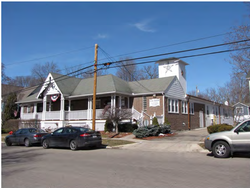
Main West 520_Looking Northwest
