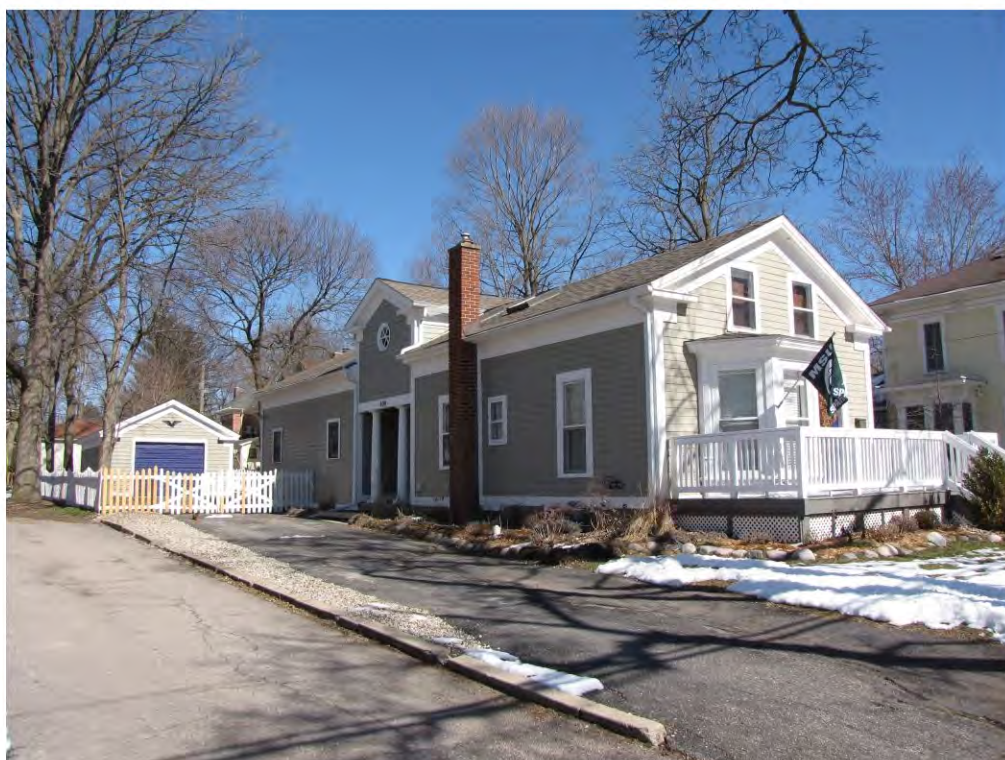
Main West 508_Looking Northeast
